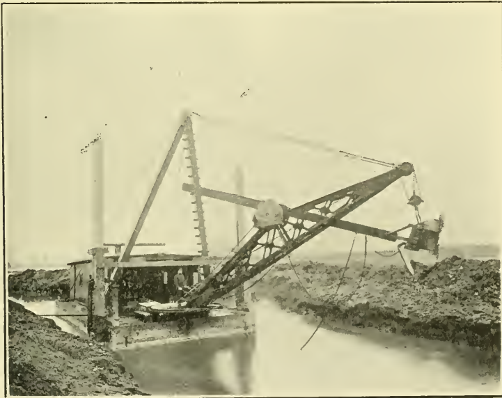
Fig. 5.—1-yard Bucyrus dredge.—Coldwater Portland Cement Co.
