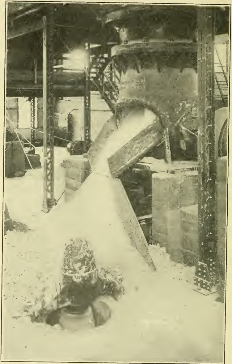
Fig. 19.—Crushers—Tidewater Portland Cement Co. (One No. 9 and two No. 6 gyratory crushers).
