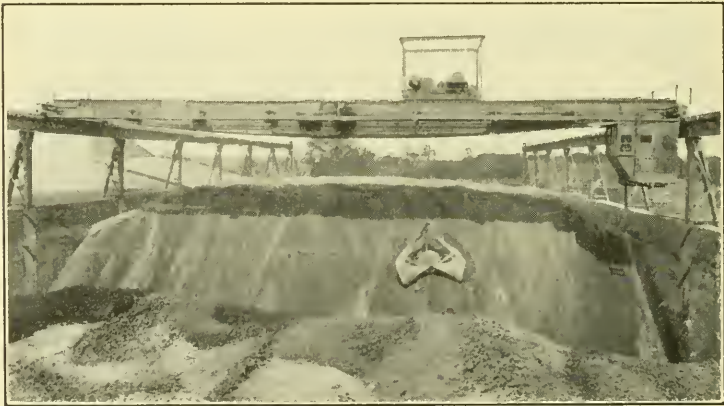
Fig. 114.—Clinker handling bridge crane, 80 ft. span, at the Bath Portland Cement Co., Shepard Electric Crane and Hoist Co., maker.
