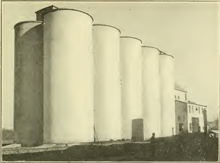
Fig. 119.—Silo bins and pack house, National Cement Co., Montreal, Que.
