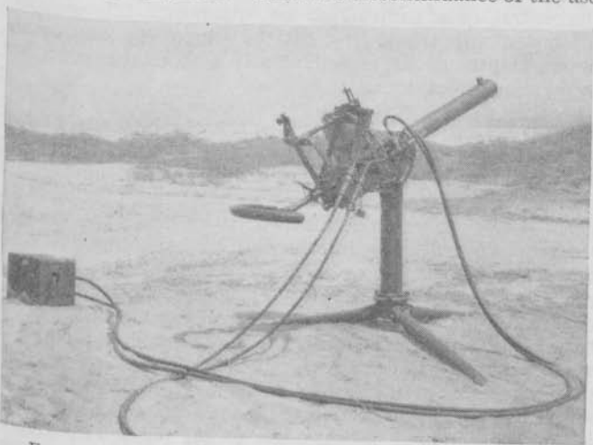
FIGURE 54.—M2 mount with central tracer control sighting equipment.
