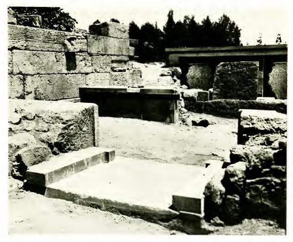
FIG. 180. VIEW THROUGH DOORWAY OF ENTRANCE HALL SHOWING 'COURT OF STONE SPOUT' WITH BALUSTRADE AND GYPSUM ORTHOSTAT OF WALL BEYOND.
