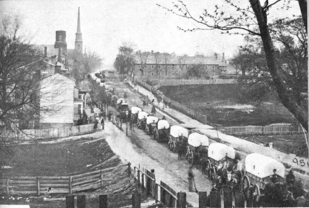
In 1864 nearly 4,000 wagons traveled with Meade's Army of the Potomac, each capable of carrying 2,500 pounds of supplies. During one year the Federal Army purchased 14,500 wagons and captured an additional 2,000.
