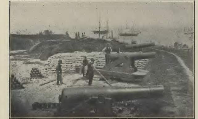
THE CONFEDERATE COMMAND OF THE RIVER. (Battery Magruder, Yorktown.) Looking north up the river, four of the five 8-inch Columbiads composing this section of the battery are visible. The grape-shot and spherical shells, which had been gathered in quantities to prevent the Federal fleet from passing up the river, were abandoned on the hasty retreat of the Confederates, the guns being spiked. The vessels in the river are transport ships, with the exception of the frigate just off shore.
