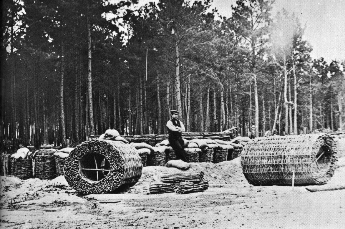
Gabions, open-end baskets filled with earth, proved as effective as masonry in defensive works. Thousands of these baskets were patiently made by hand for use in field and seacoast fortifications.
