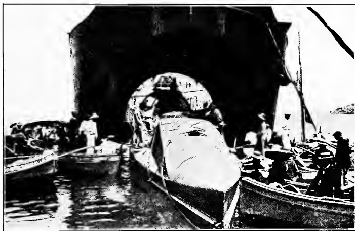
Submarine entering through the open bow construction
