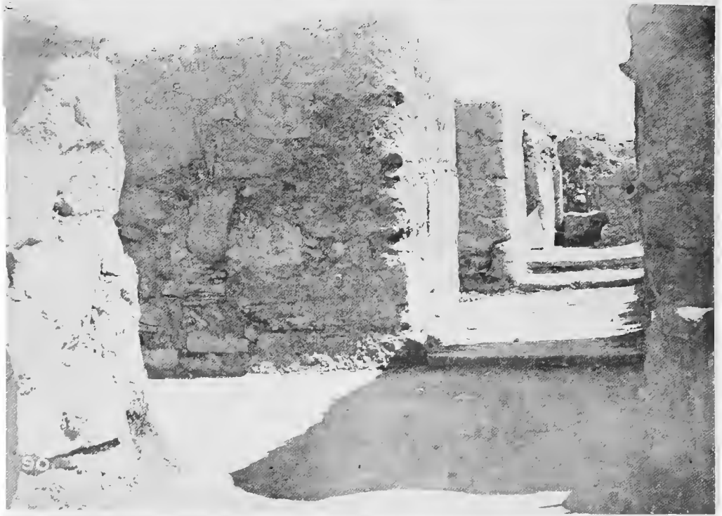
FIG. 277. CORRIDOR OF BAYS SHOWING PIERS THAT ACTED AS SUPPORTS FOR FRONTAL PILLARS OF EAST HALL ABOVE.
