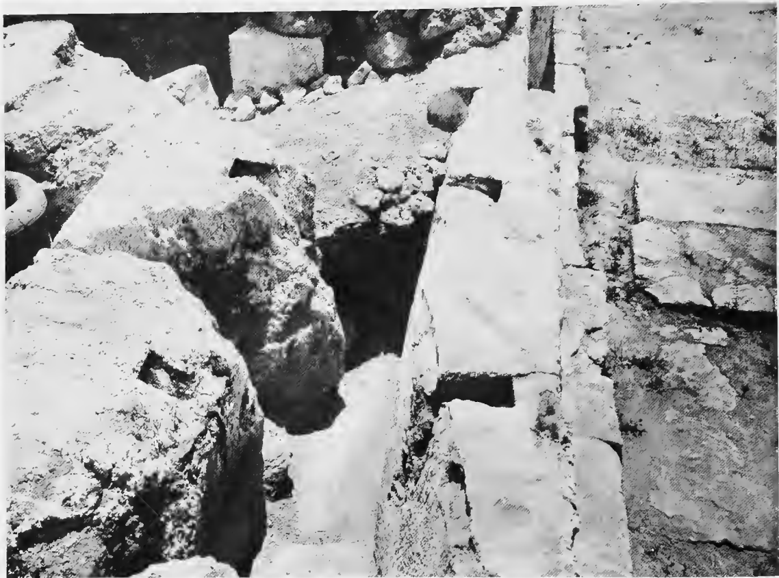
FIG. 95. VIEW SHOWING INTERIOR OF W. WALL, KNOSSOS, WITH PART OF THE RUBBLE FILLING REMOVED. MORTISES FOR WOODEN CROSS-BARS ARE VISIBLE.
