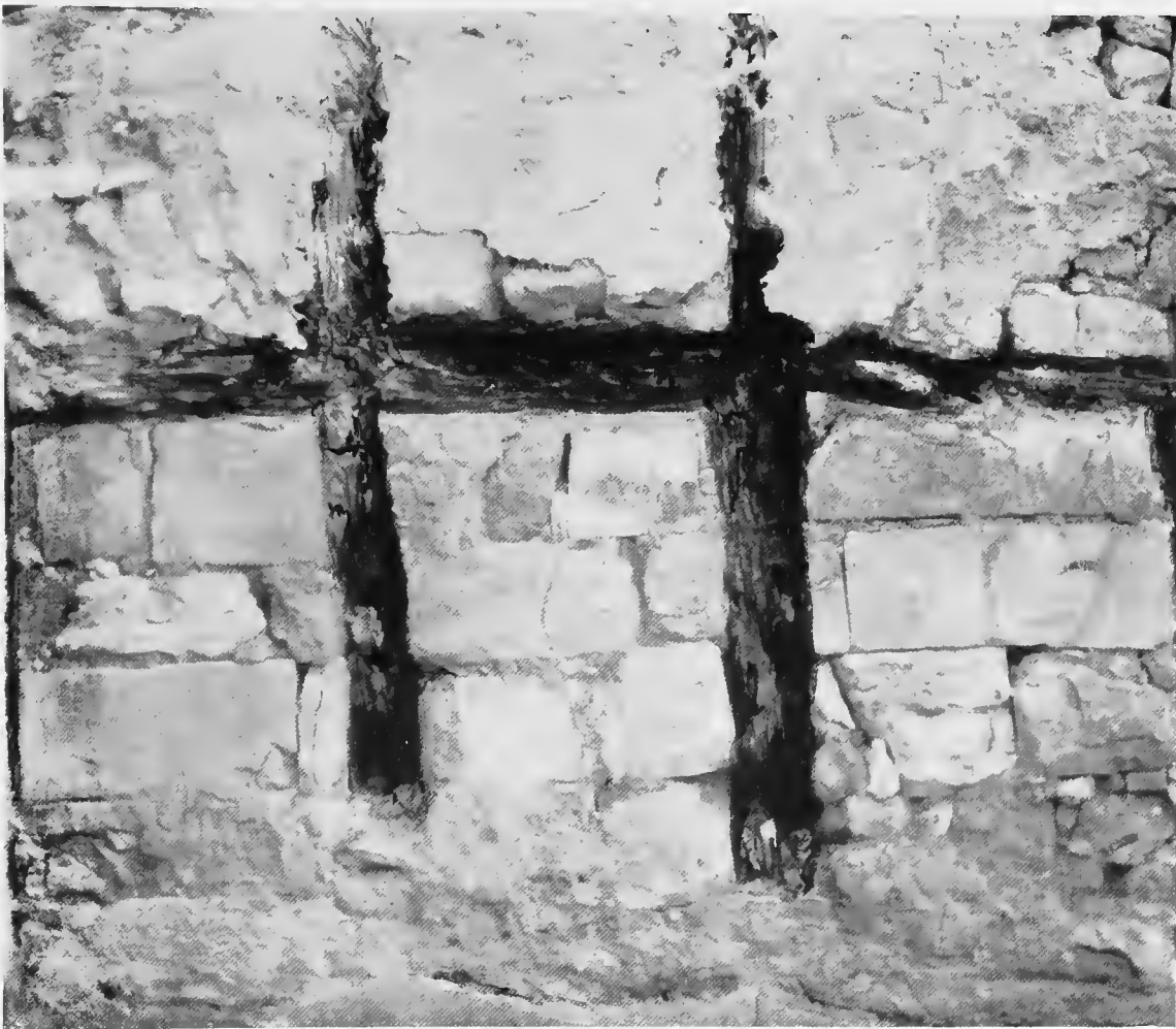
FIG. 251. PART OF S. WALL OF 'HALL OF DOUBLE AXES' SHOWING TIMBER FRAMEWORK. BROKEN EDGE OF GYPSUM WAJNSCOTING BELOW.
