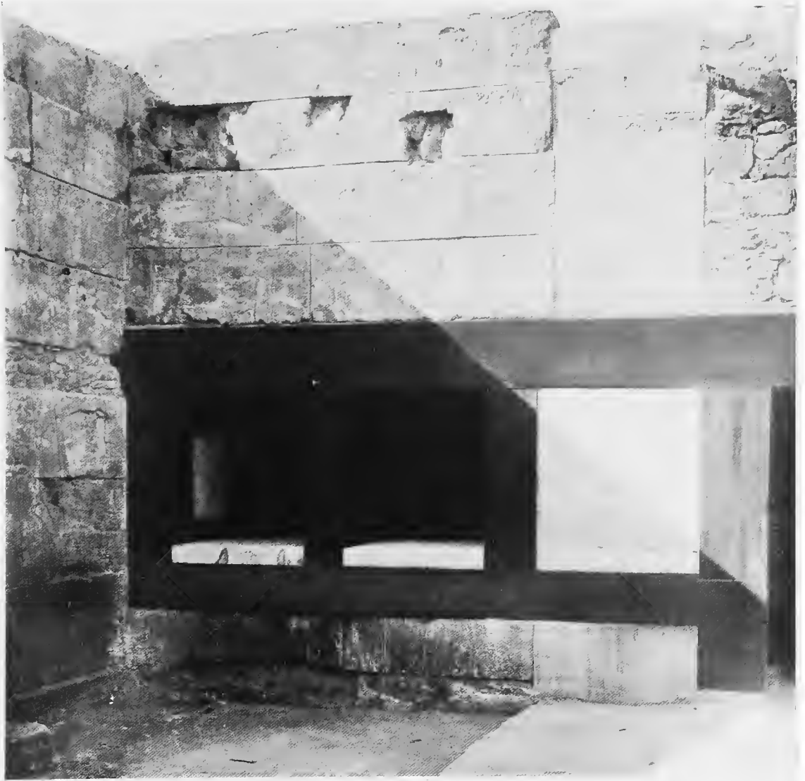
FIG. 253 b . WINDOW NORTH OF W. LIGHT-AREA OF HALL, AS RESTORED, WITH THE MASONRY ABOVE RAISED TO ITS ORIGINAL POSITION.
