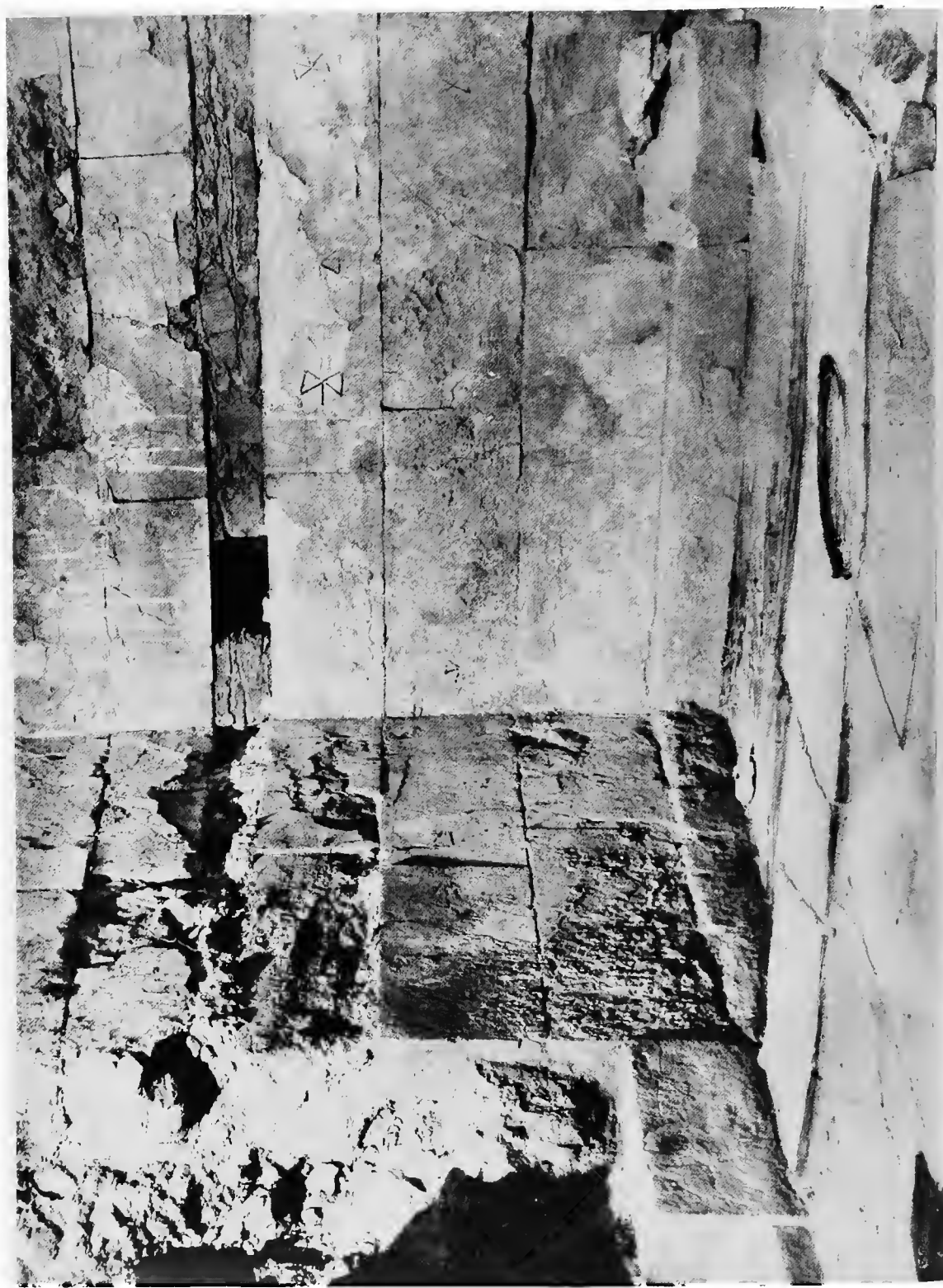
FIG. 250. S.W. ANGLE OF LIGHT-WELL, HALL OF DOUBLE AXES SHOWING PART OF STYLORATE (THE GAP IN THE MASONRY LEFT BY THE DECAY OF THE STYLORATE), AND OTHER PART OF THE WALL.
