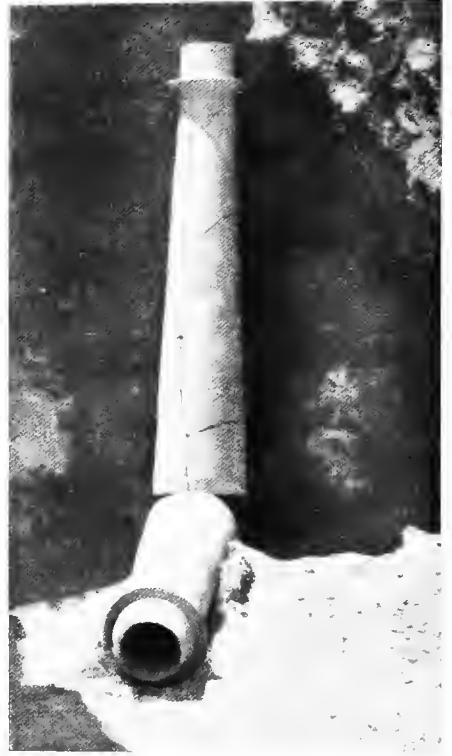
FIG. 103. CLAY WATER PIPES: NEAR AREA OF STONE DRAIN-HEAD.
