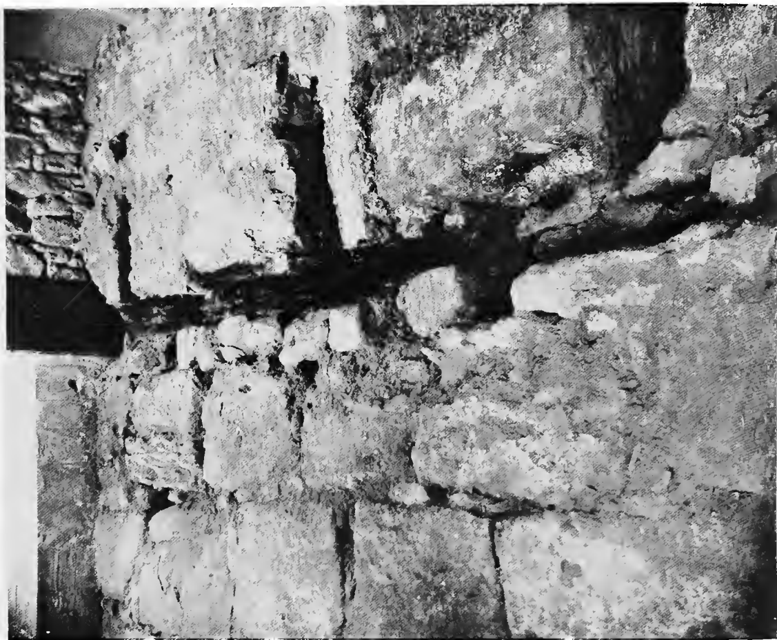
FIG. 252. WALL OF 'LOWER E.-W. CORRIDOR' SHOWING TIMBER FRAMEWORK AND INTERVENING PIERS, SUPERIMPOSED ON EARLIER MASONRY.
