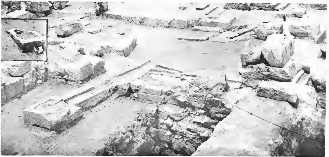
FIG. 275. STONE DRAIN-HEAD AND CONDUIT. (INSET, SMALLER DRAIN-HEAD.)
