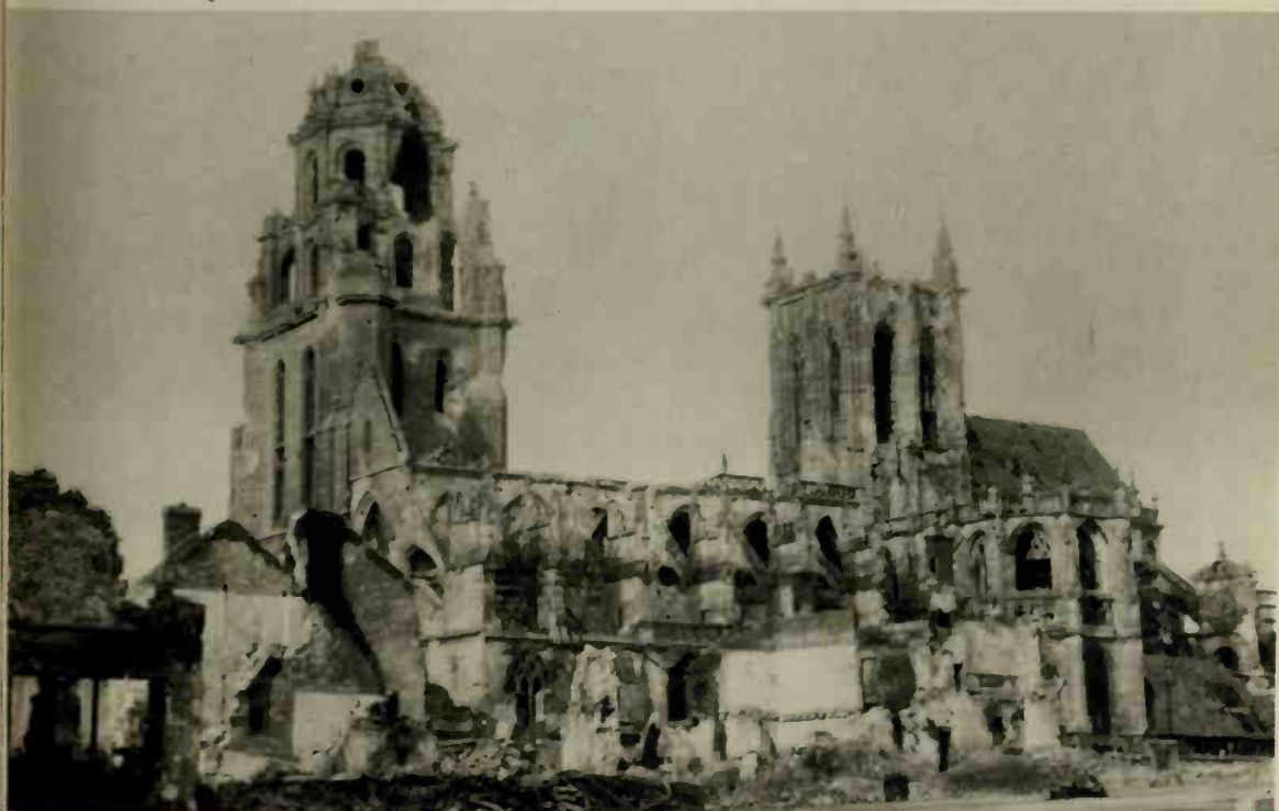
253. Argentan: Church of Saint-Germain in Ruins Argentan: Eglise Saint-Germain en Ruines
