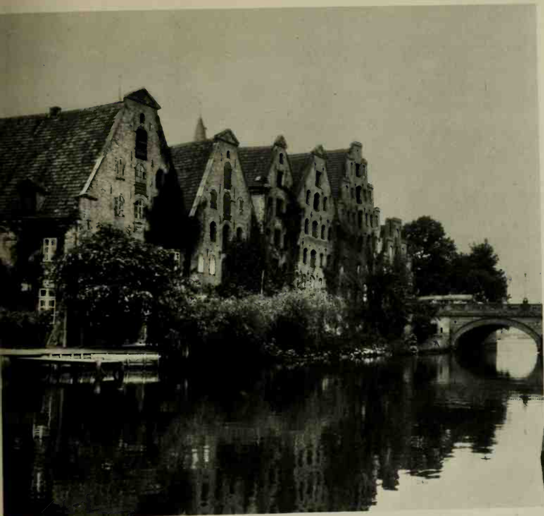
411. Lübeck: The Salt Houses (xiv century) Lubeck: Entrepôts de Sel (xive siècle)
