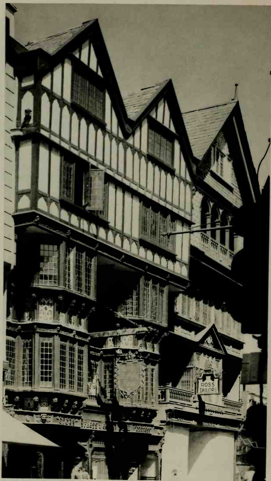
86 Exeter: Old Houses in High Street (xvi century) Exeter: Vieilles Maisons de High Street (xvii siècle)
