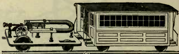
FIG. 24.—HALL LOCOMOTIVE OF 1850-1.
