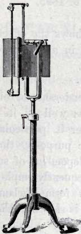
FIG. 133.—PHOTO-ENGRAVING ARC LAMP.
