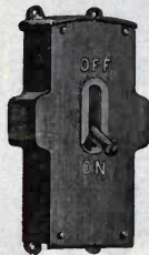
FIG. 72.—CUT-OUT SWITCH.
