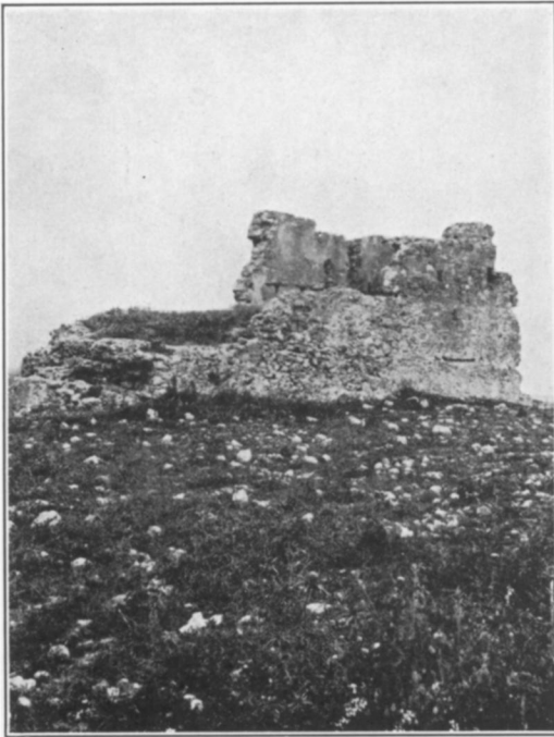
FIGURE 58. REMAINS OF LARGE BUILDING
