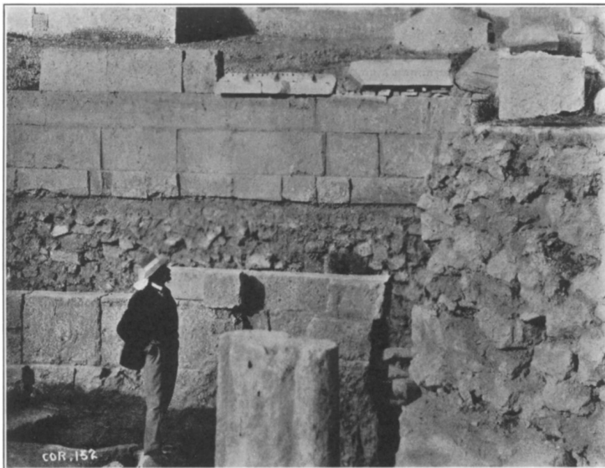
FIGURE 116. VIEW OF WEST FACE OF "GOOD HIGH WALL." THE RUBBLE FOUNDATION FOR THIS WALL APPEARS BEHIND A TERRACE WALL BELONGING TO THE ROMAN PERIOD BEFORE THE CONSTRUCTION OF THE PROPYLAEA
