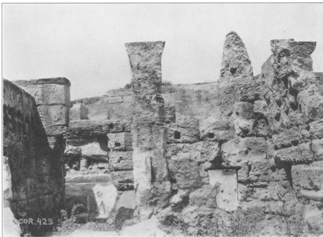
FIGURE 106. SPRING OF VAULT ON PARTITION OF WEST SHOPS ALONG LECHAEUM ROAD
