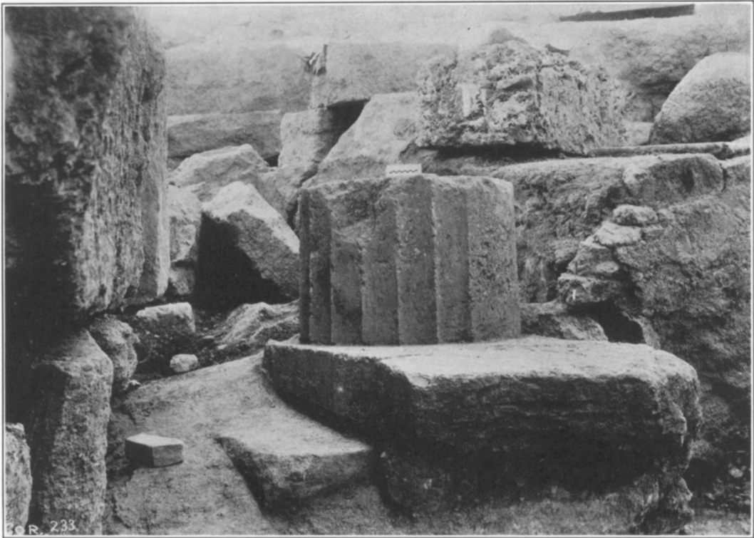
FIGURE 145. NORTH BUILDING. VIEW SHOWING COLUMN
