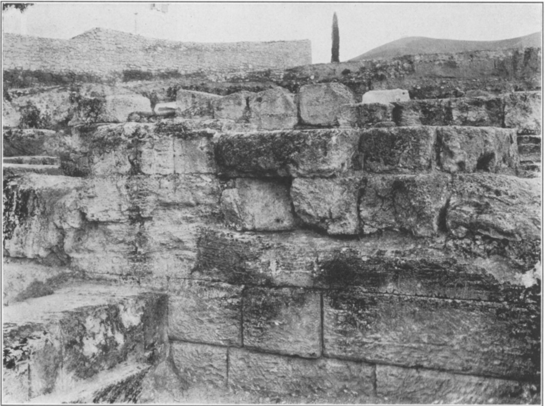
FIGURE 120. JUNCTION OF EAST WALL OF MAIN PLATFORM WITH THE EAST PYLON OF THE CENTRAL ARCH OF THE PROPYLAEA
