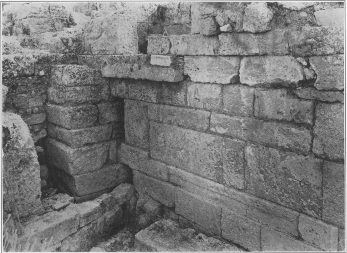
FIGURE 117. JUNCTION OF WEST BUTTRESS OF PROPYLAEA AND EPISTYLE WALL. AN EARLY ROMAN TERRACE WALL APPEARS BELOW THE BUTTRESS
