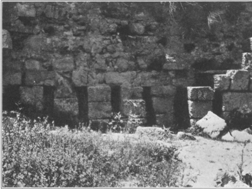
FIGURE 22. ISTHMIAN WALL WITH HOLES FOR WATER
