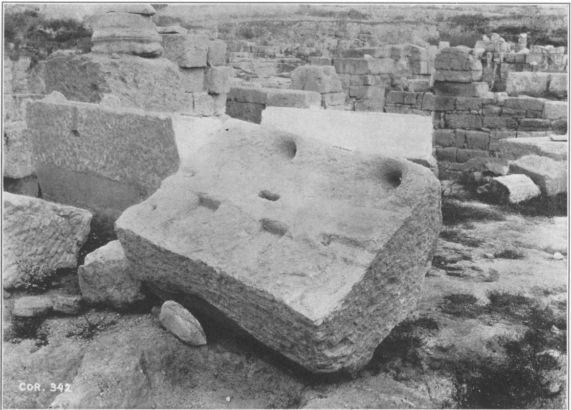
FIGURE 143. TOP VIEW OF CORNICE SHOWN IN FIGURE 142
