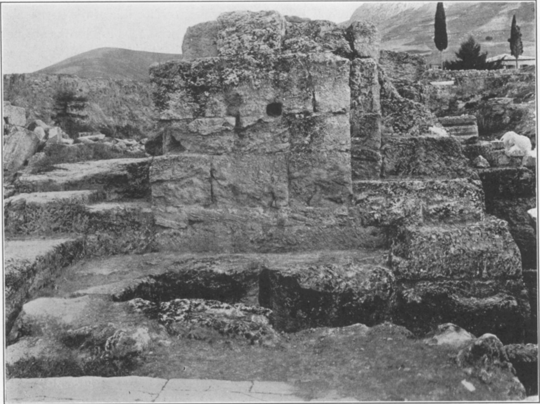
FIGURE 118. WESTERN PIER OF CENTRAL ARCH OF PROPYLAEA
