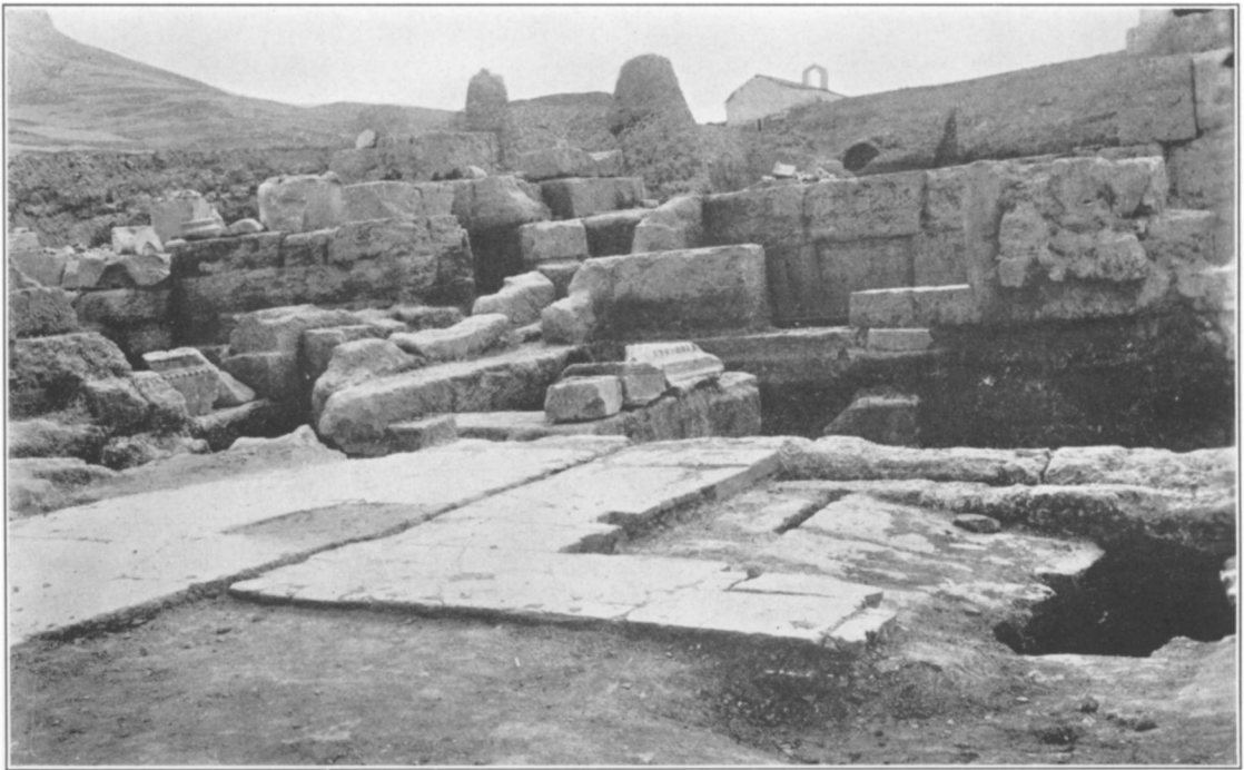
FIGURE 115. MAIN PLATFORM OF PROPYLAEA. THE HOLE AT THE RIGHT WAS MADE BY THE EXCAVATORS TO REACH THE COMPLEX OF DRAINS UNDER THE PLATFORM
