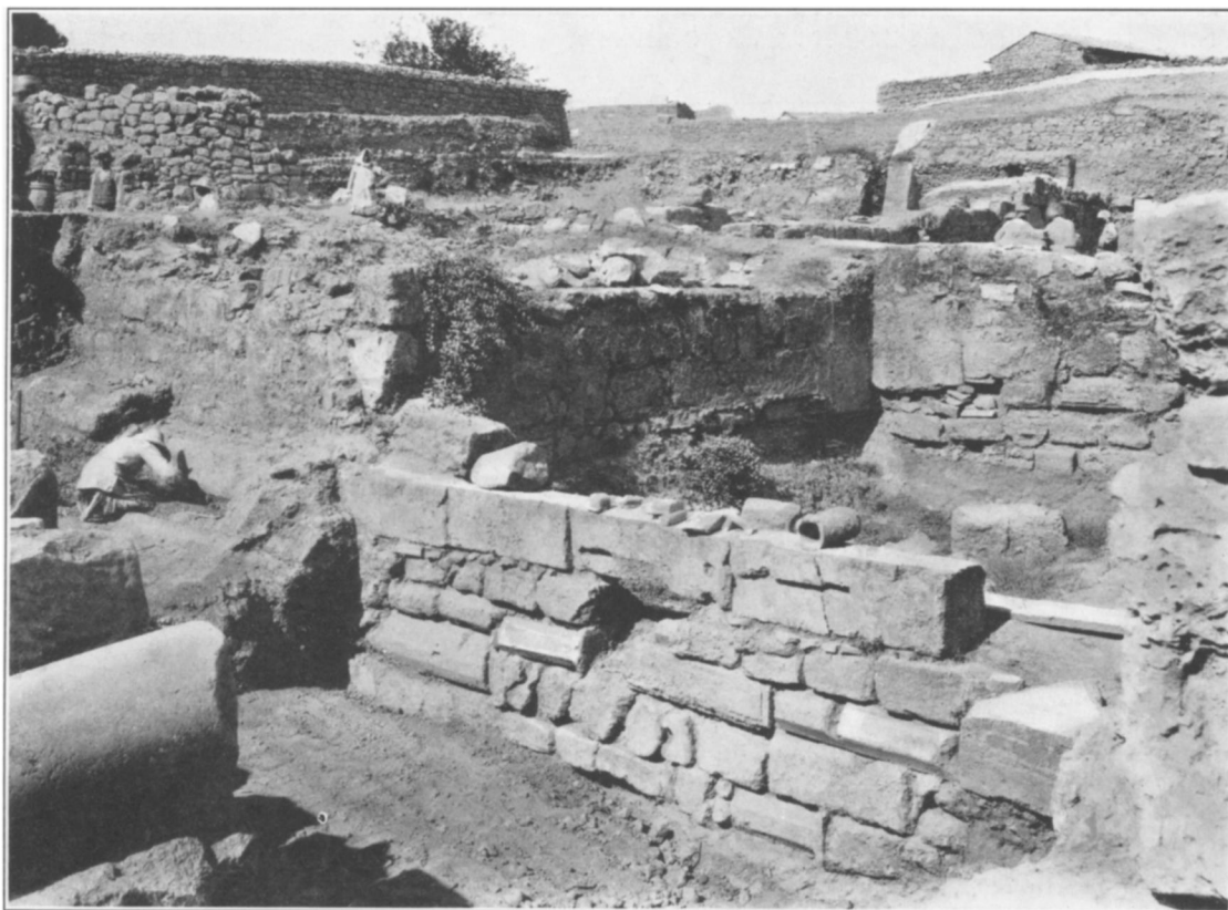
FIGURE 109. EAST SHOPS. FOUNDATION OF SHOP FRONT WALL, SHOWING RE-USED GREEK MATERIAL
