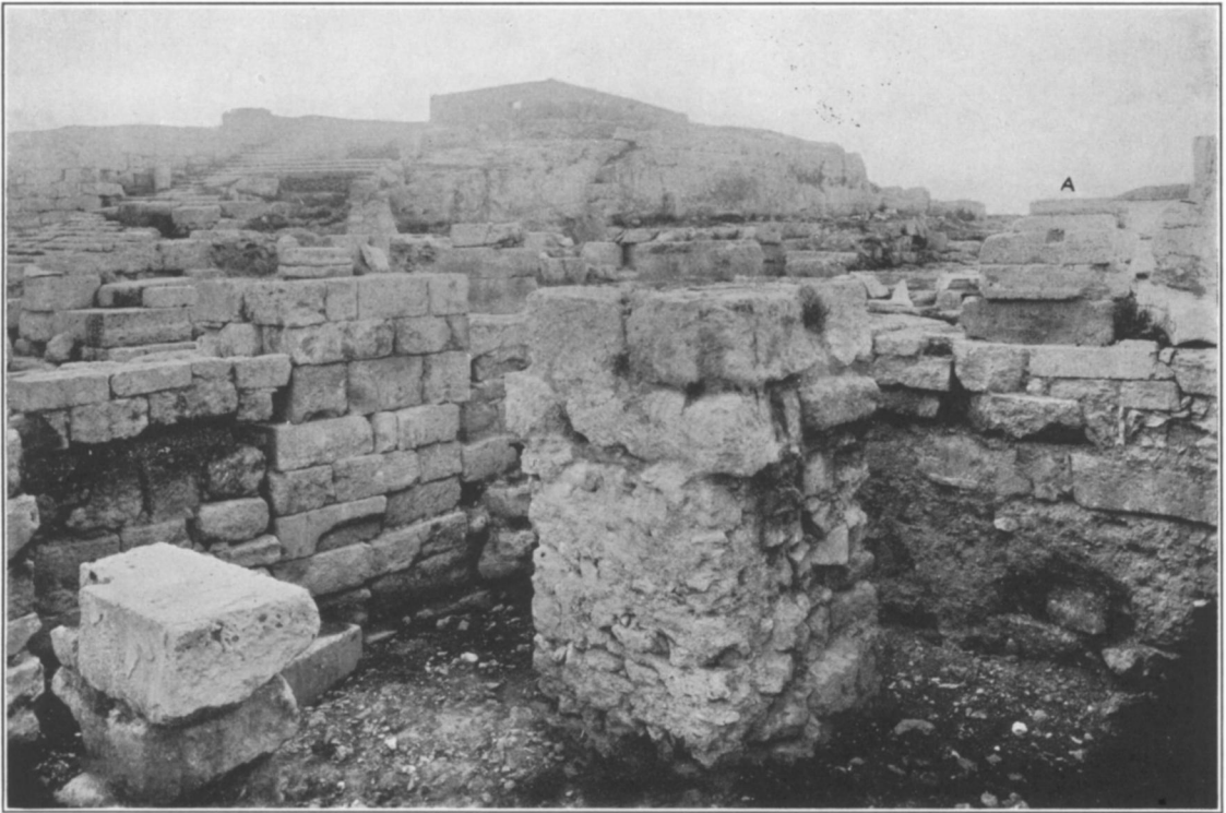
FIGURE 132. FOUNDATION PIERS FOR INTERIOR COLUMNS AT SOUTH END OF LATER BASILICA
