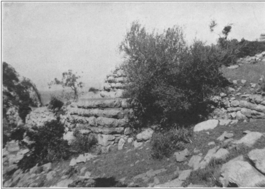
FIGURE 10. OENOË: SOUTHWEST TOWER
