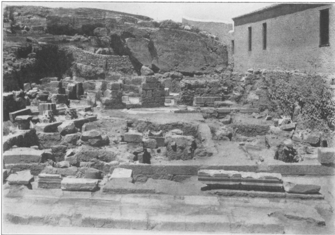
FIGURE 101. AREA NORTH OF BASILICA. VIEW LOOKING WEST
