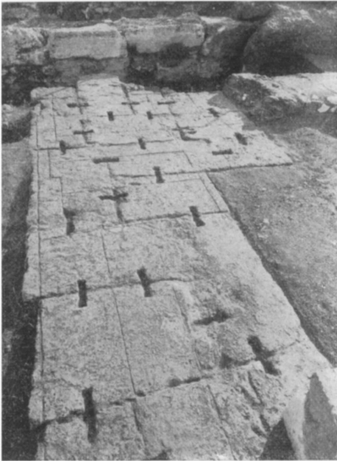
FIGURE 22. N. E. CORNER OF SCENE-BUILDING, SHOWING SETTING LINES ON TOECHOBATE
