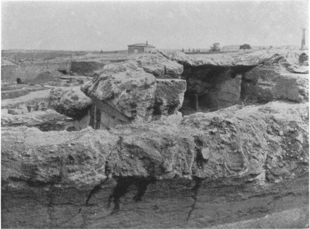
FIGURE 18. HORIZONTAL VAULT BELOW WEST VOMITORIUM (LEFT) AND SLOPING VAULT (RIGHT) TO THE SOUTH
