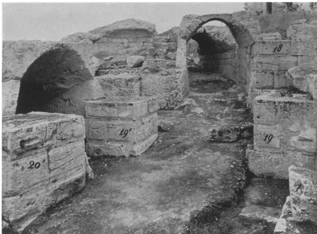
FIGURE 9. WEST END OF SEMICIRCULAR CORRIDOR
