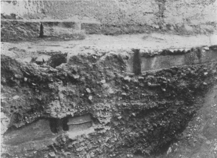
FIGURE 12. FOUNDATION FOR OUTER WALL OF CAVEA, SOUTHEAST SIDE
