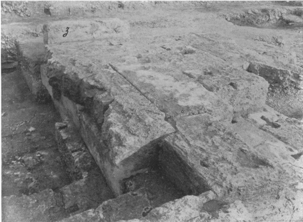
FIGURE 29. TRACES OF STAIRS, WEST OF STAGE
