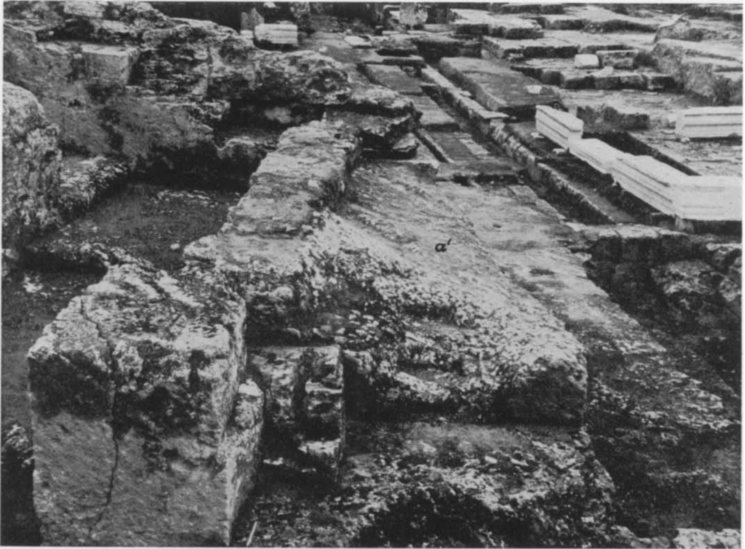
FIGURE 2. EARLY ROAD NORTH OF EAST STAIRWAY
