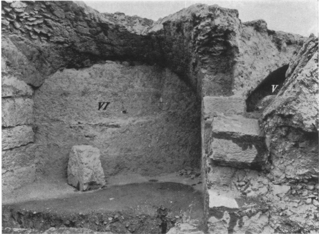
FIGURE 19. VAULTS OVER CHAMBERS V AND VI, SHOWING DIFFERENCE IN SLOPE
