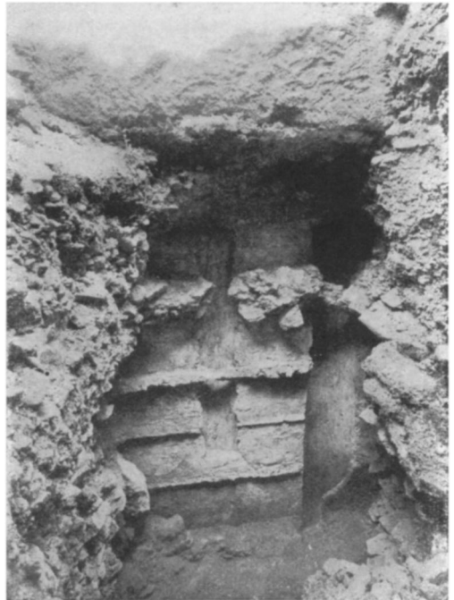
FIGURE 21. FOUNDATION FOR OUTER WALL OF CAVEA, SOUTH SIDE
