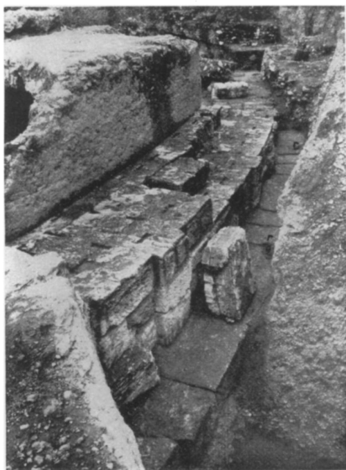
FIGURE 14. OUTER WALL OF CAVEA AND VAULT OVER SEMICIRCULAR CORRIDOR, SOUTHWEST SIDE
