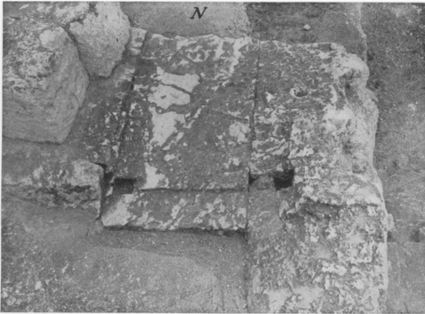
FIGURE 35. TRACES OF THE DOOR BETWEEN ROOM N AND THE ARENA
