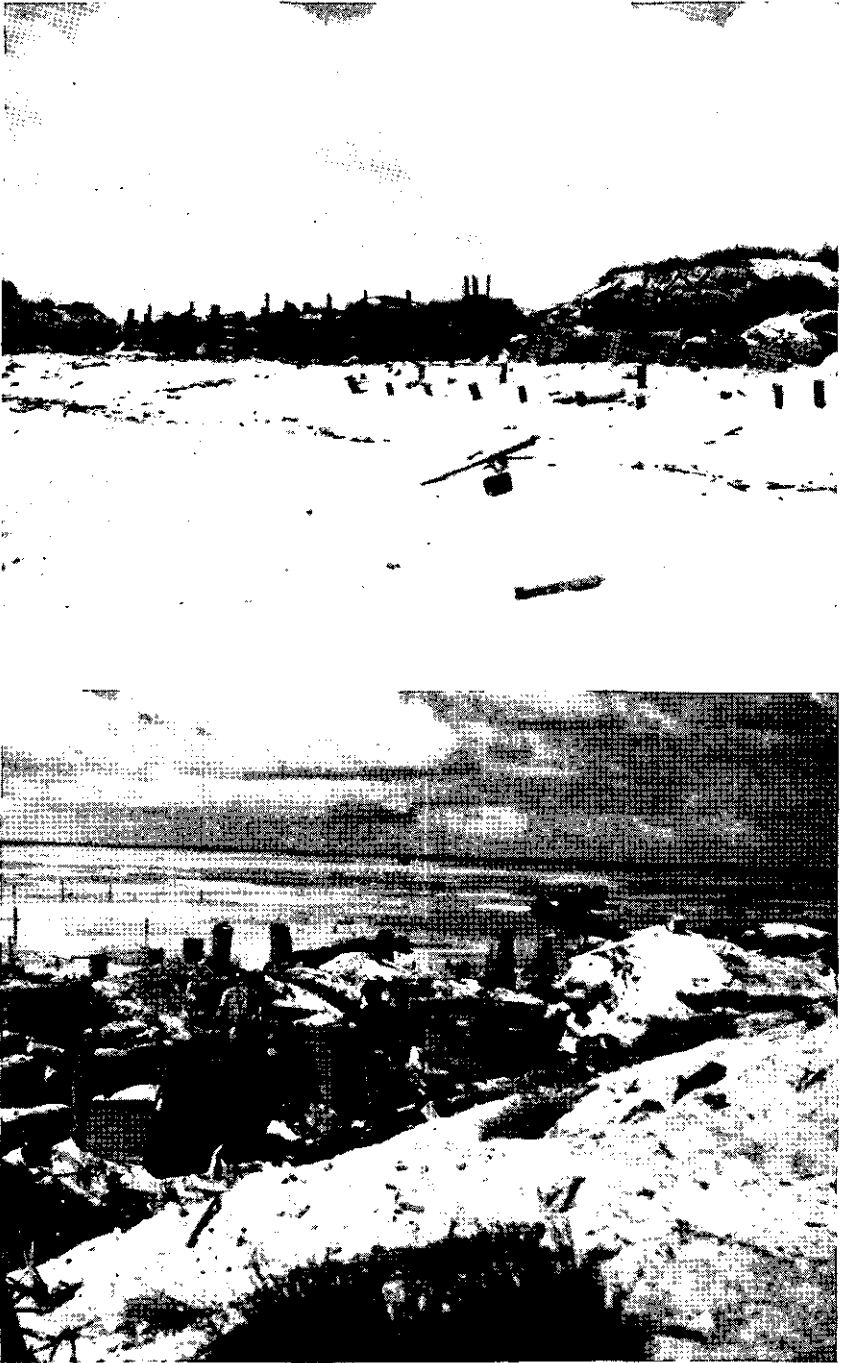
Figure 10.—Portion of sea wall on Betio (above); Japanese barricade positions behind sea wall (below).
