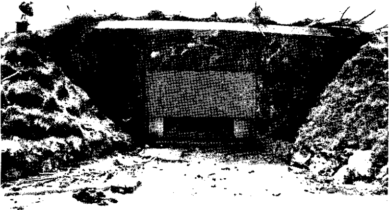
Figure 28 (b).—Closeup of the circular pillbox shows the steel embrasure lining and cover.
