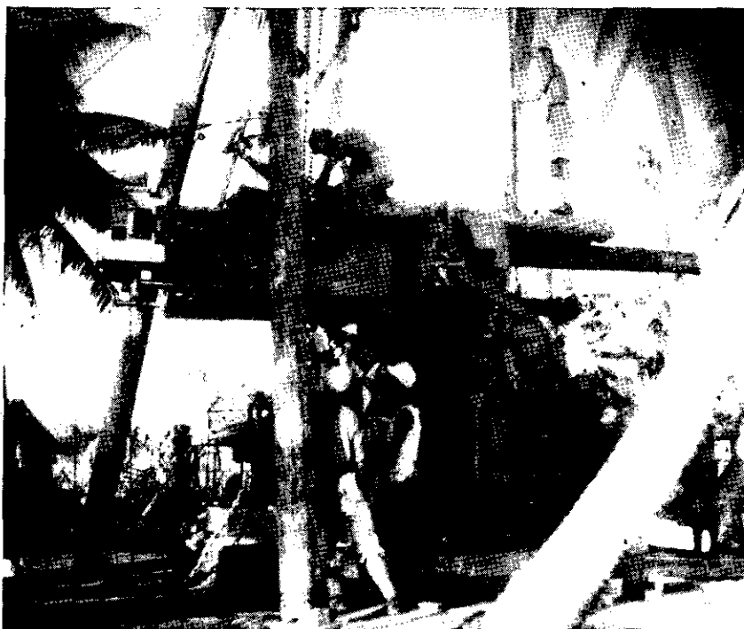
Figure 59.—Installing one gun of a twin-mount 127-mm Model 89 gun.
