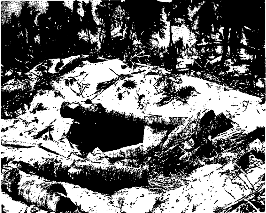
Figure 34.—Gunport in Japanese log and sand pillbox on Betio.
