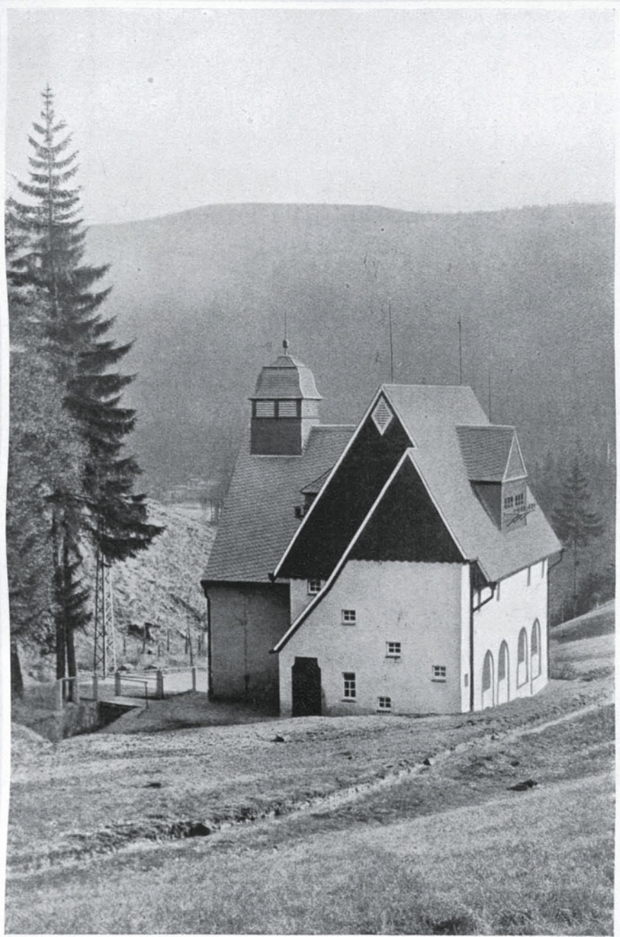
Transformatorstation Blauenthal (E. W. Obererzgebirg)
