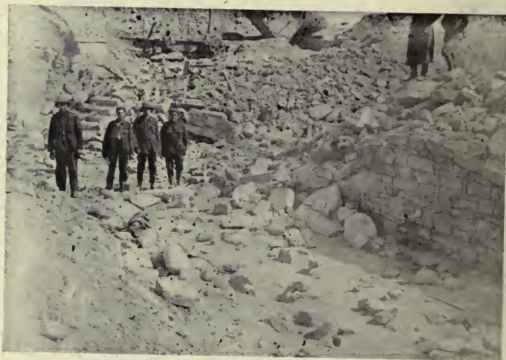
1. EXTERIOR OF SEDD-UL-BAHR FORT.
