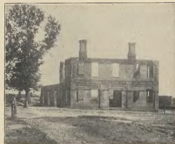
THE SOUTH CAROLINA RAILROAD OFFICES
