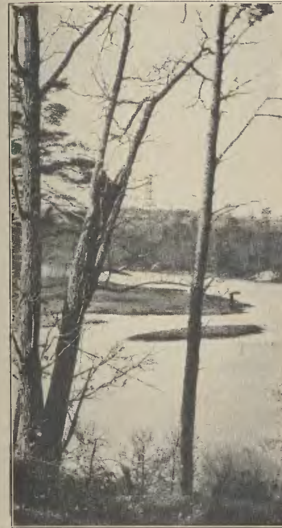
BUTLER'S SIGNAL TOWER
