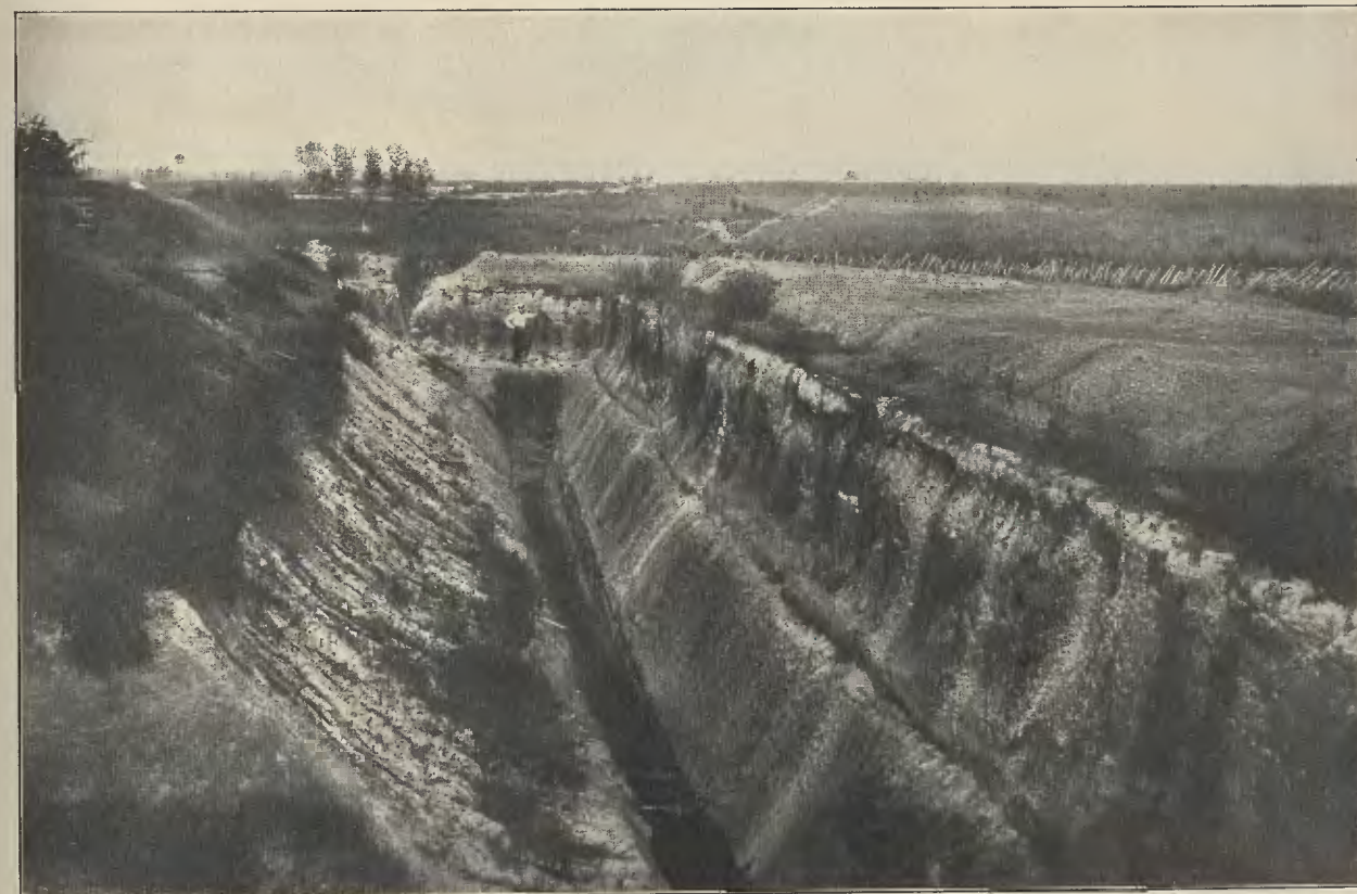
THE 27-FOOT DITCH AT FORT GILMER, GUARD AGAINST FEDERAL MINES
