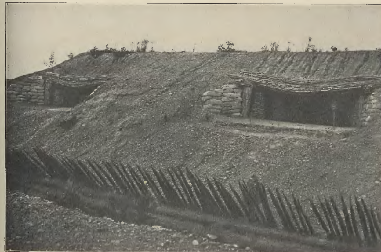
PALISADES AND PARAPET AT FORT HARRISON
