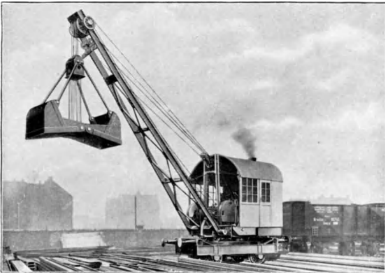
Fig. 3. Steam slewing crane
