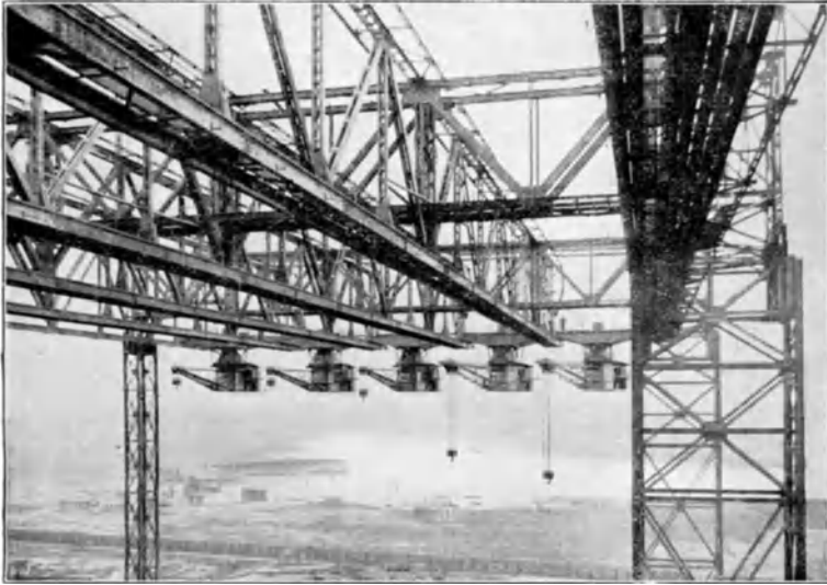
Fig. 37. Five slewing cranes suspended from overhead runways
