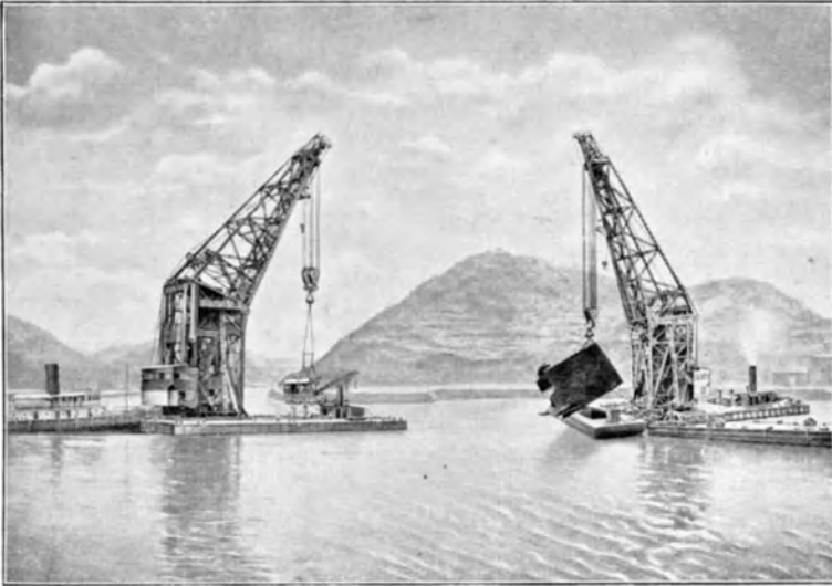
Fig. 41. Giant floating crane employed in the Panama Canal
