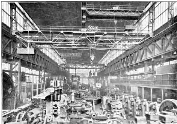
Fig. 9. Travelling cranes for the work shop running one above the other
