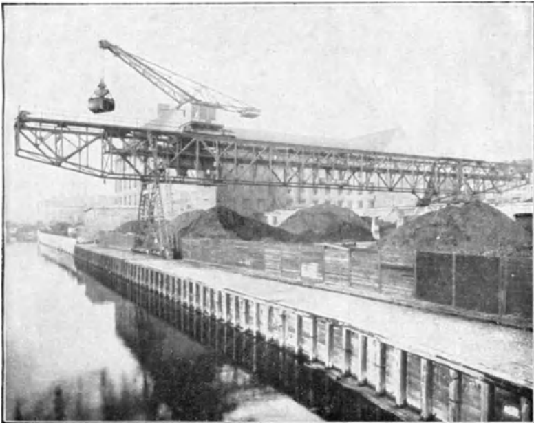
Fig. 25. Loading bridge with travelling slewing crane
