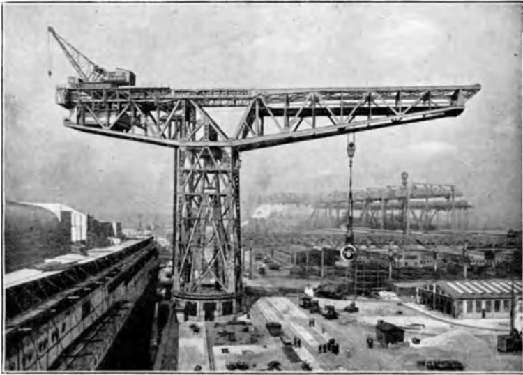
Fig. 39. Hammer head crane with slewing crane, crab and luffable jib
