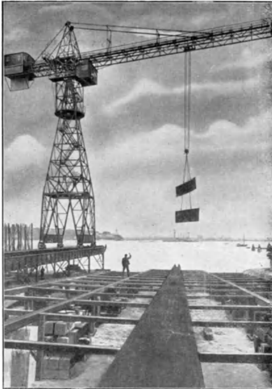
Fig. 36. Travelling turret slewing crane
