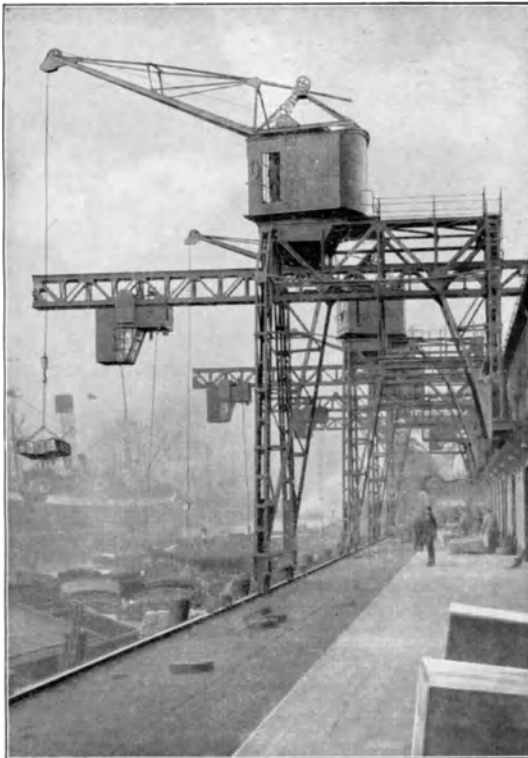
Fig. 32. Double crane with crab and slewing crane
