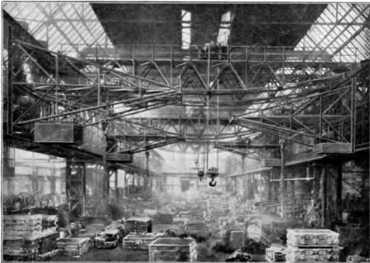
Fig. 18. Travelling bracket crane
