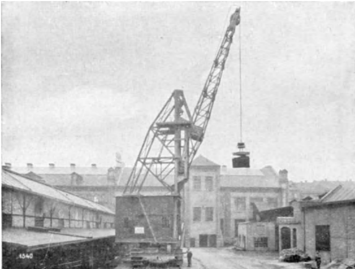
Fig. 34. Luffing crane with raised jib
