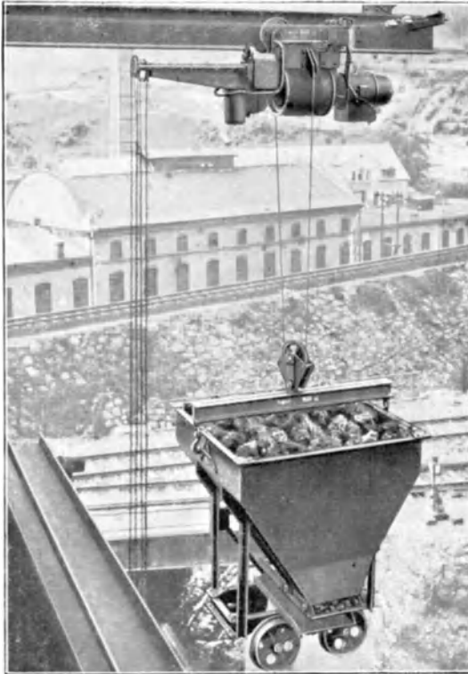
Fig. 24. Electric block transporting coal trucks
