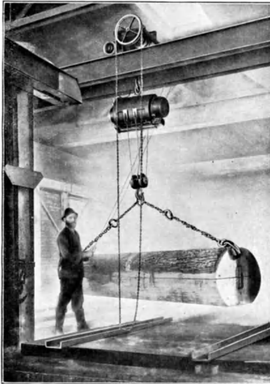
Fig. 5. Electric block pulley
