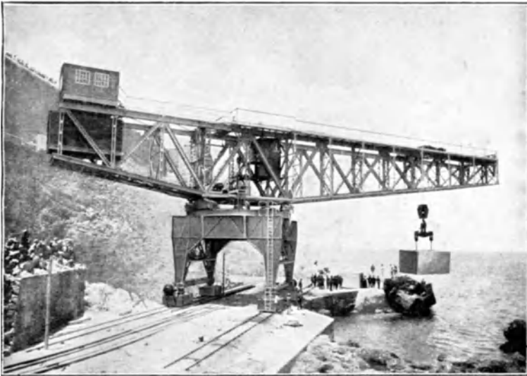
Fig. 7. Electrically driven jib-crane
