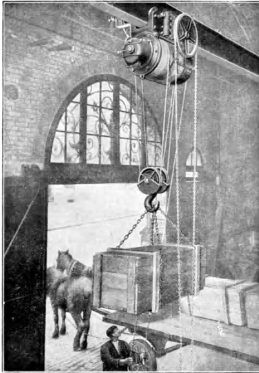
Fig. 6. Travelling electric block
