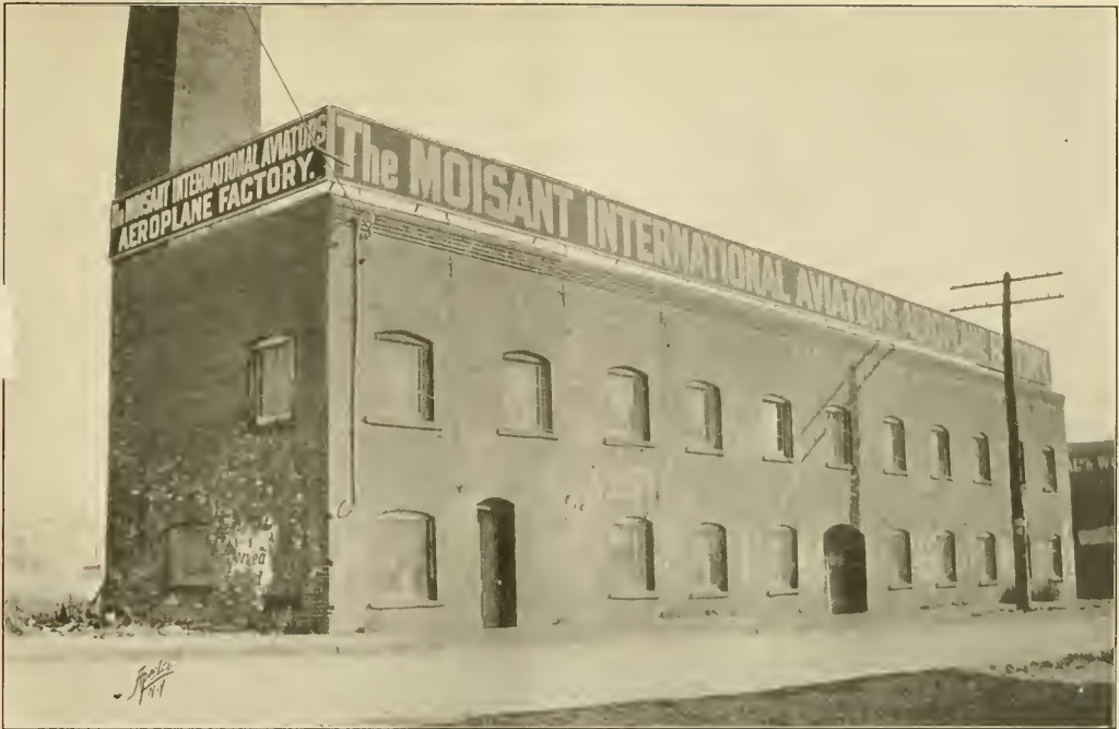
The above picture is a reproduction of the Moisant Aeroplane Factory on Long Island. In these works all of the Moisant Monoplanes have been constructed up to the present time. Harold Kantner is now in charge of this factory.
