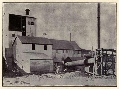
FIG. 76. - DRYING FURNACE, PLANT NO. 2, SULPHIDE CORPORATION.
