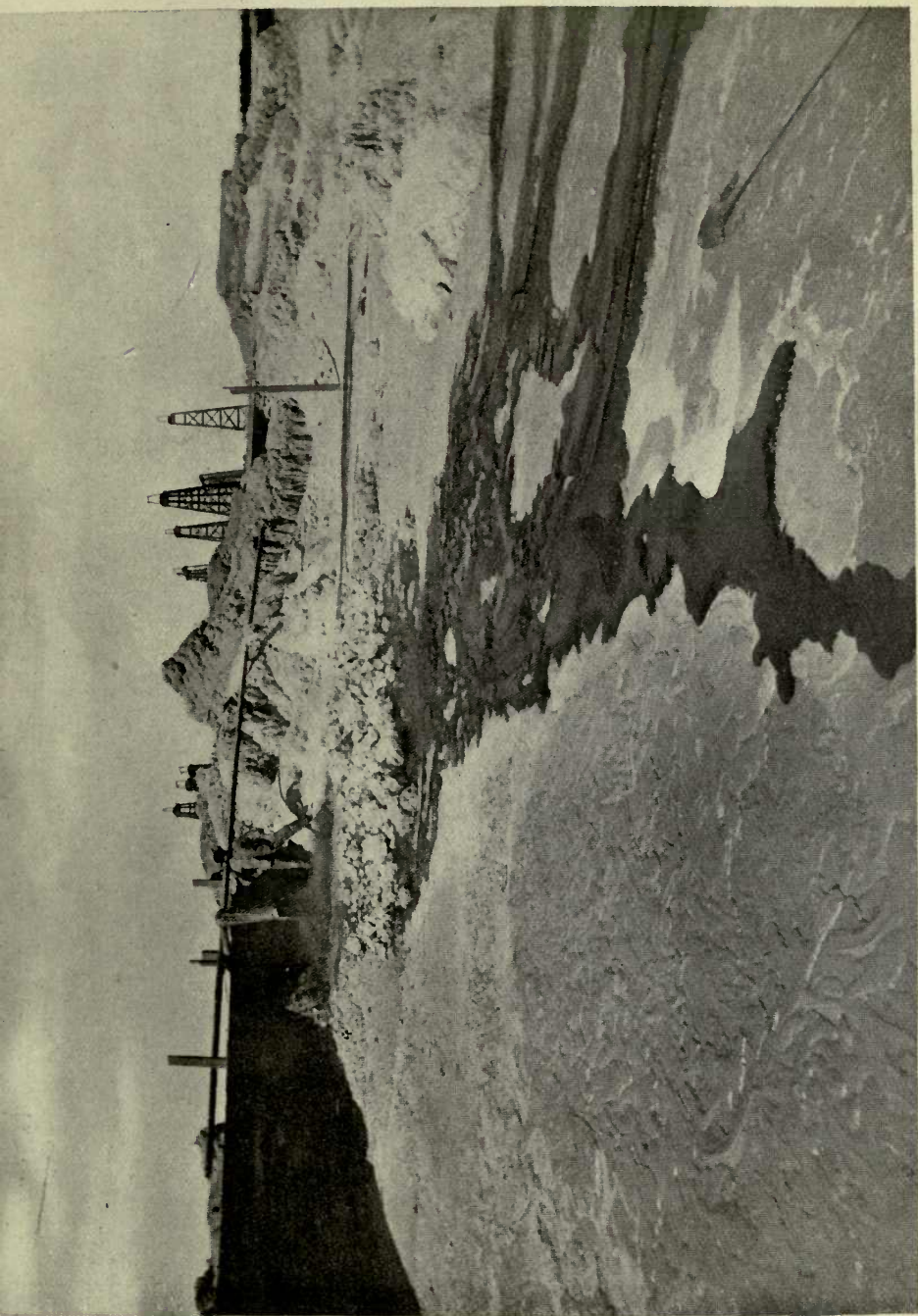
LOUISIANA SULPHUR MINES. Filling up a bin (a block) fifty feet high.
