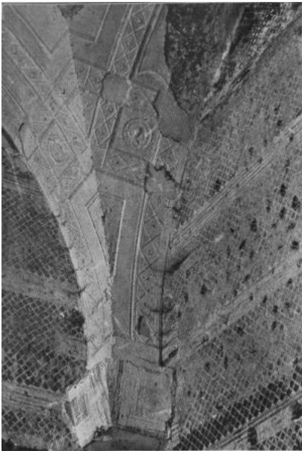
Photo. Moscioni OPUS RETICULATUM FROM THE THERMAE OF HADRIAN'S VILLA AT TIVOLI
