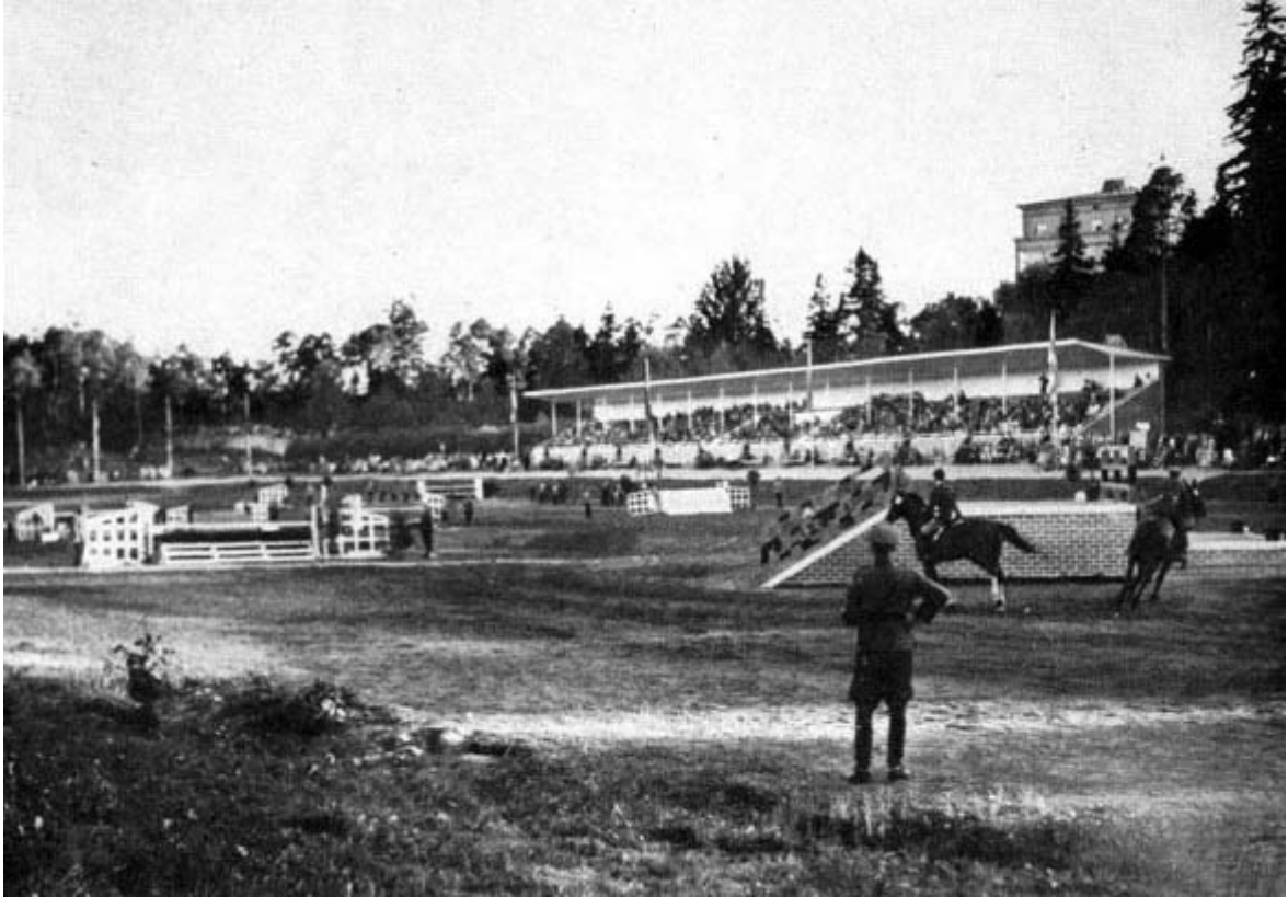
The Laakso riding grounds and roofed stand.
