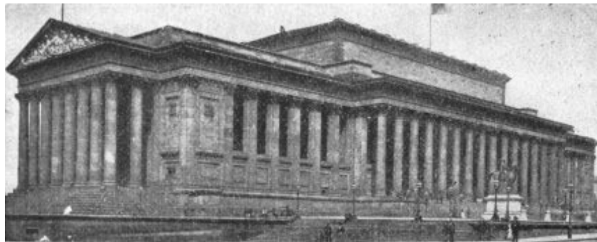
FIG. 199.—ST. GEORGE'S HALL, LIVERPOOL.
