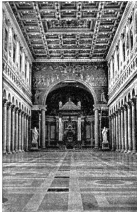
FIG. 68.—ST. PAUL BEYOND THE WALLS. INTERIOR.
