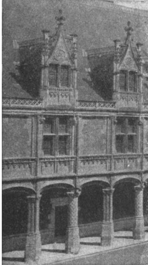
FIG. 175.—BLOIS, COURT FAÇADE OF WING OF LOUIS XII.
