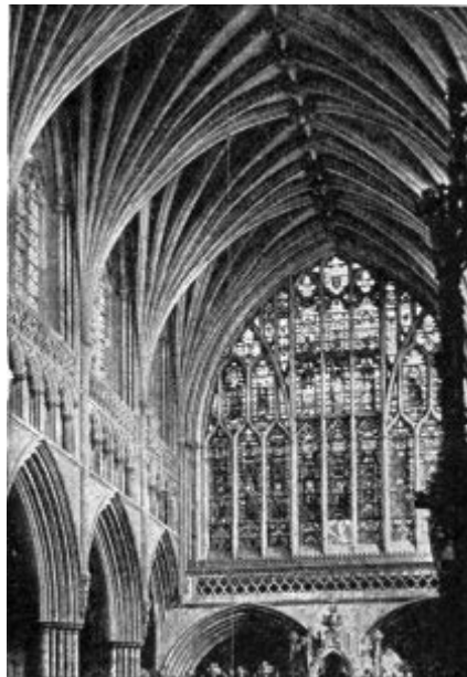
FIG. 129.—RIBBED VAULTING, CHOIR OF EXETER CATHEDRAL.
