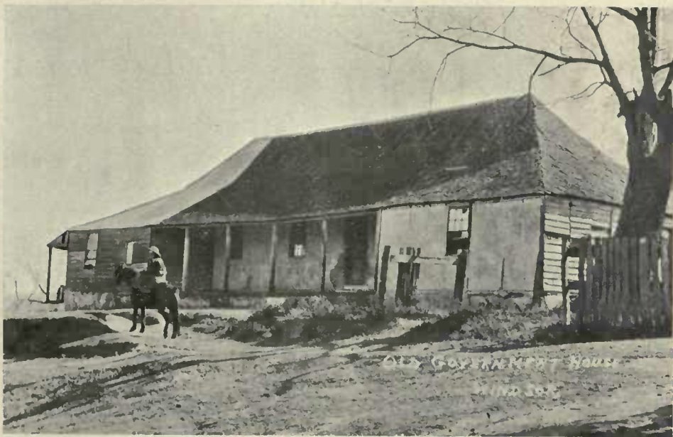
It was in the neighbourhood of Windsor—the Hawkesbury—that the first Cabinet Timber of Australia was obtained, viz., “Red Cedar,” and this is probably the house—erected about 1796—in which it was first used. The floors, skirtings, mantelpieces, doors, windows, and even the weatherboards were made of this timber and these are all in a good state of preservation to-day, 1913.
