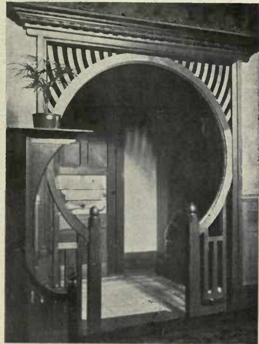
Hall Grille of Tasmanian Oak. C. B. Brady's Residence, Launceston.
