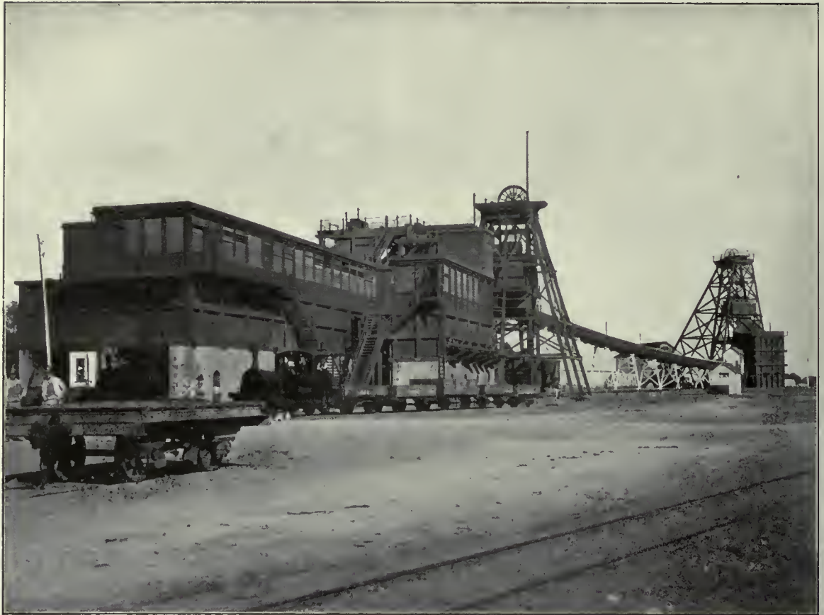
Crushing and Sorting Plant, Wallaroo Mines
