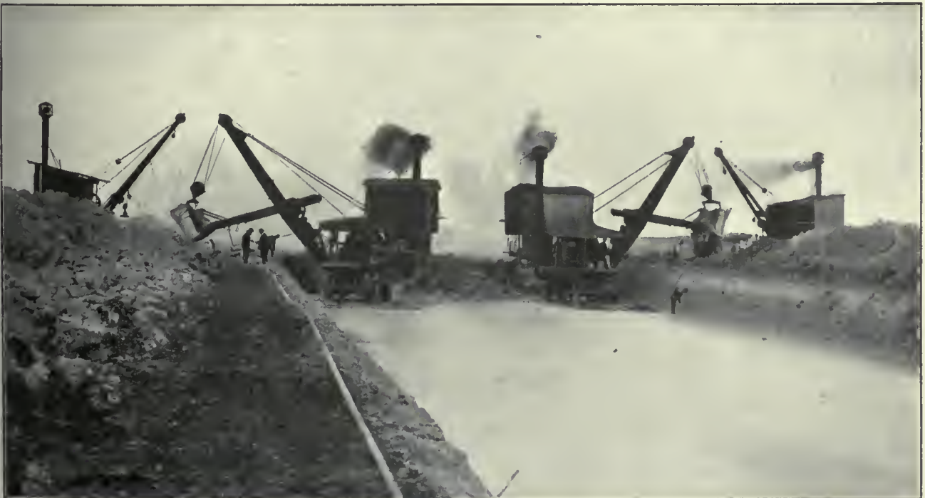
Steam Shovels at Work on South-Eastern Drains.
