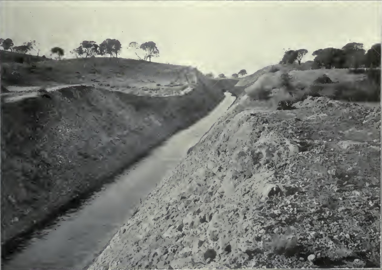
IN A NEW SOUTH WALES IRRIGATION AREA.
