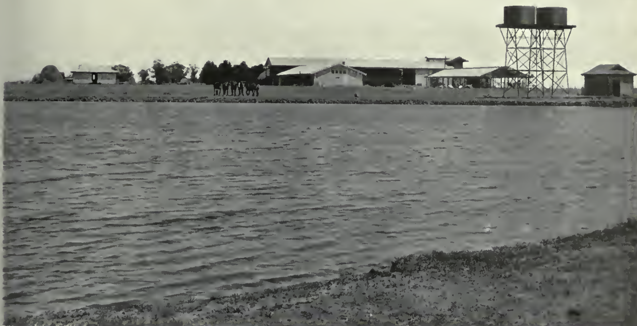
Buildings and Water Supply, State Research Farm, Werribee.
