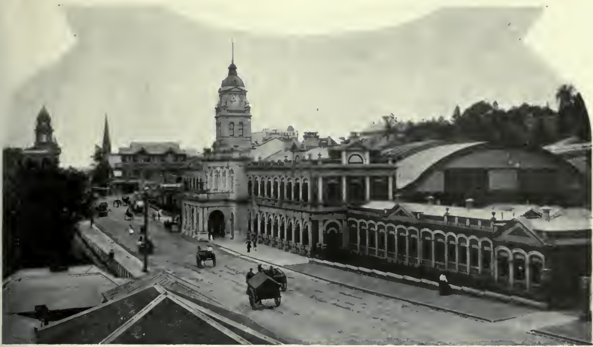
Central Railway Station, Brisbane
