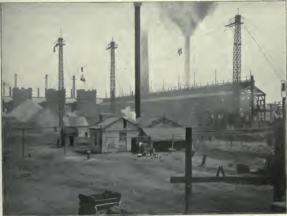
Smelting Works at Port Pirie
