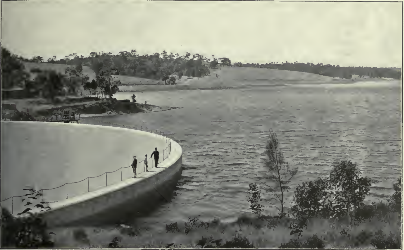
Barossa Reservoir (capacity—1,000,000,000 gallons)
