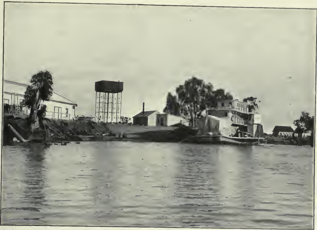
Pumping Plant at Renmark, South Australia.
