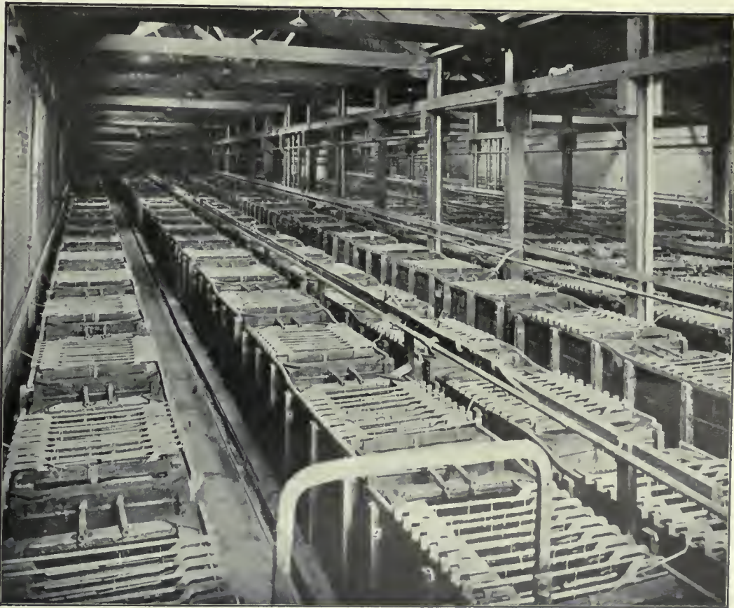
Electrolytic Room, Cobar Copper Works, N.S.W.
