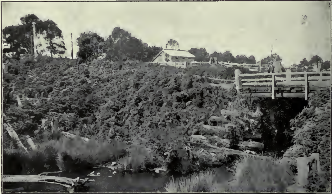
On the North Coast Road
