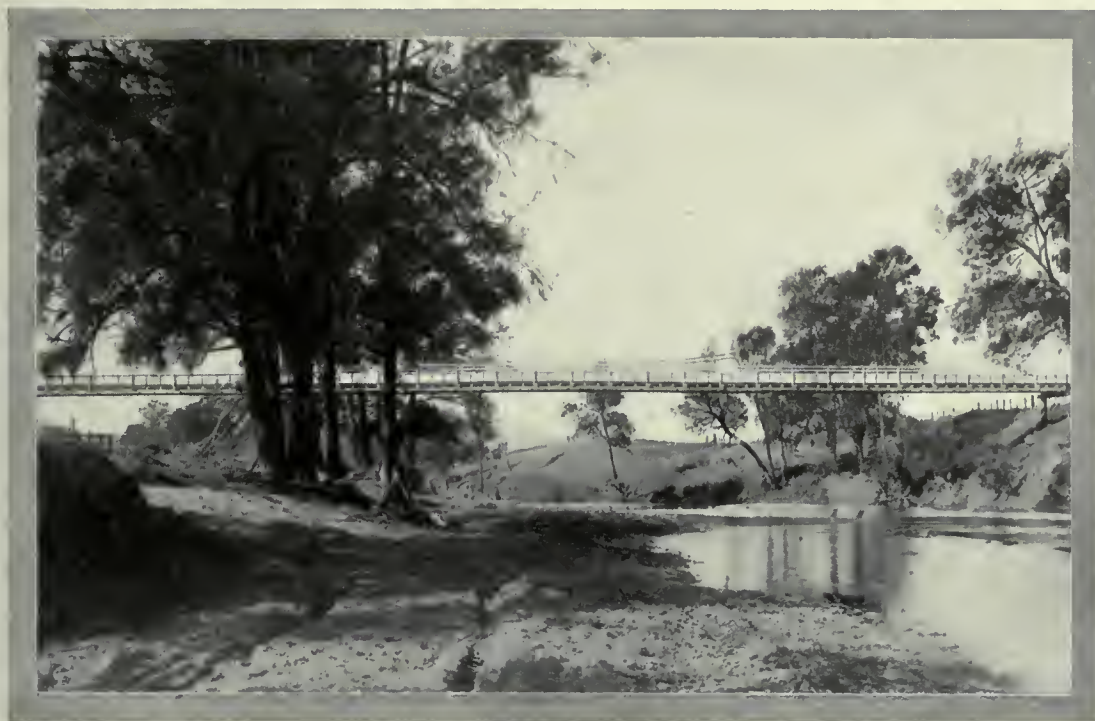
Private Suspension Bridge at Belltrees
