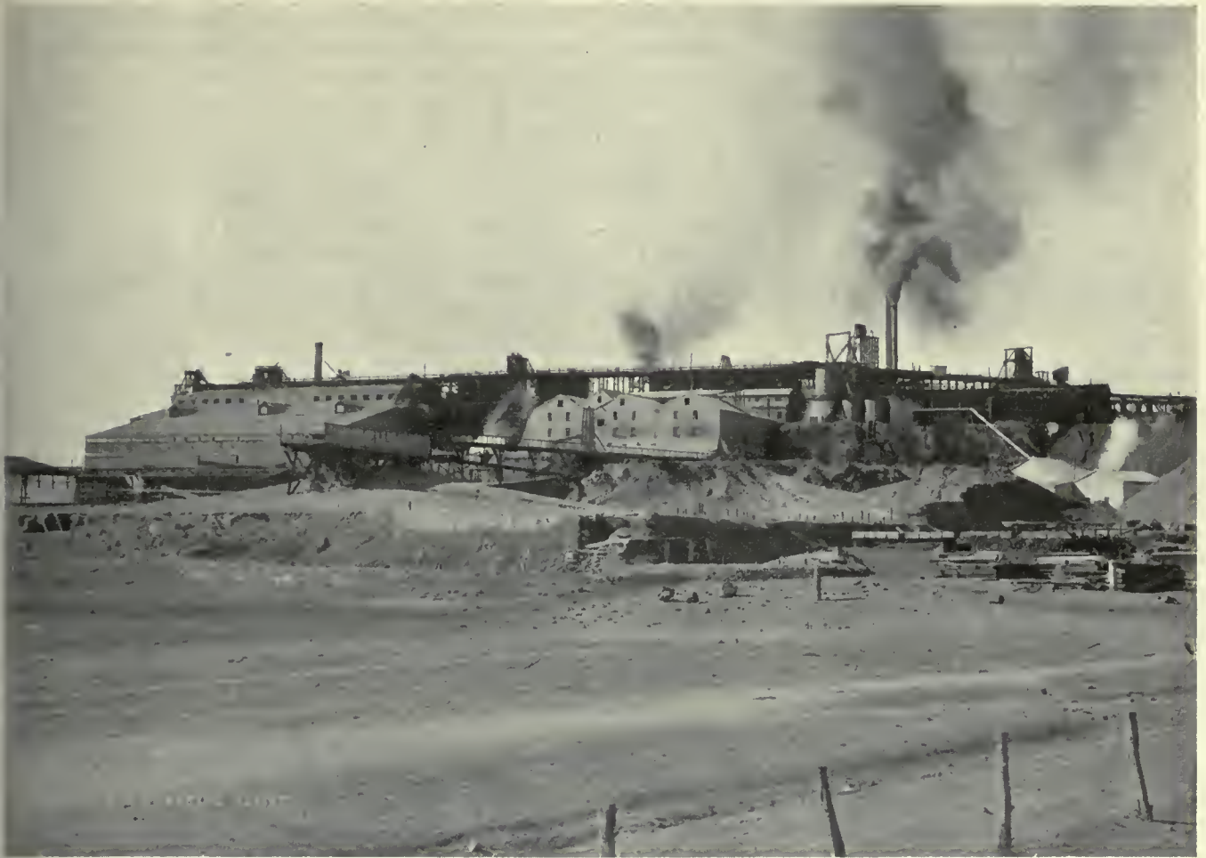
Ore Dressing Plant, Broken Hill Proprietary
