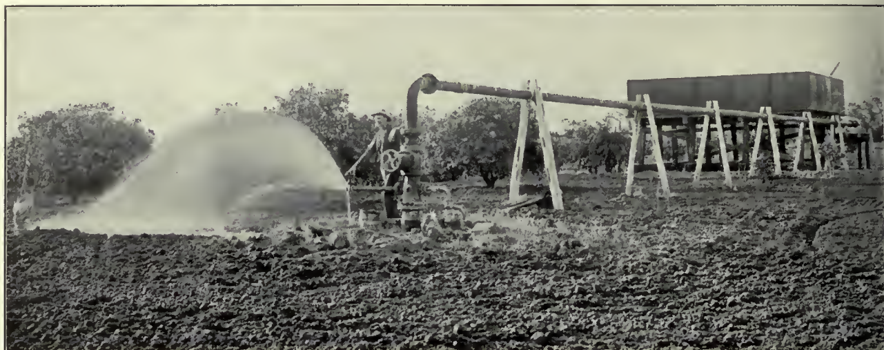
The Bore at Pera
