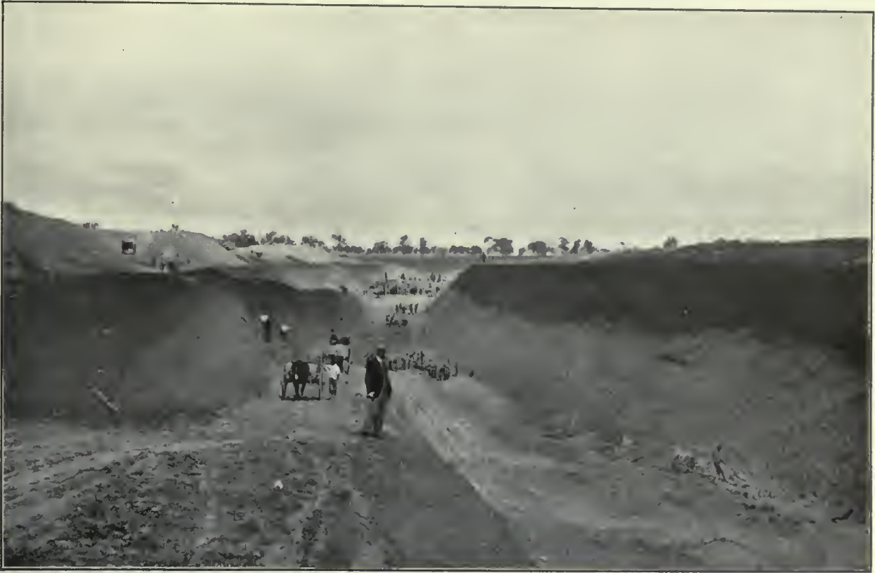
Excavation for the Waranga-Mallee Channel, Victoria
