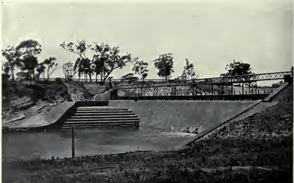
Laanecoorie Weir, on the Loddon River
