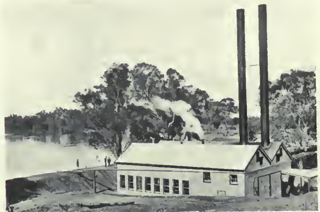
Pumping Station, River Murray
