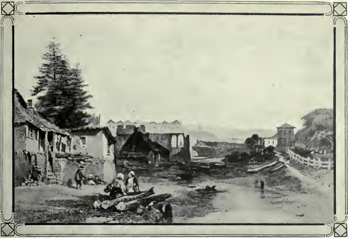
The Old Tank Stream at Sydney Cove (From a Contemporary Print)
