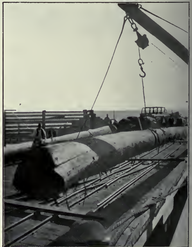
Unloading Jarrah Piles, Cossack
