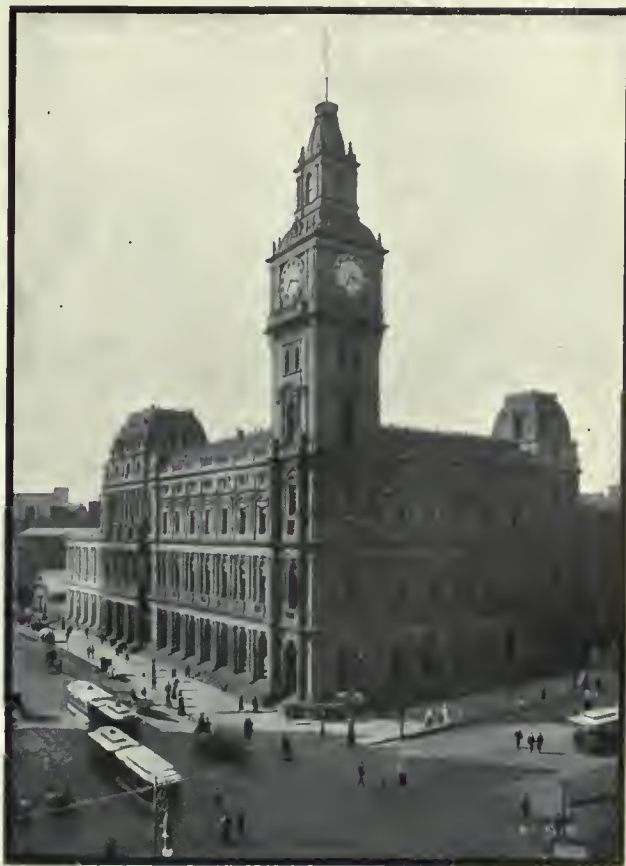
General Post Office, Melbourne
