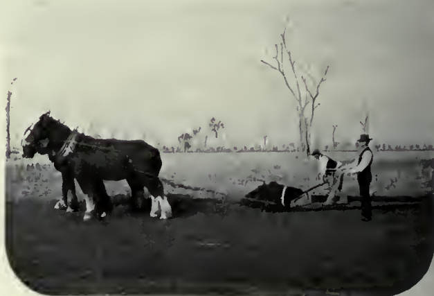
Grading Land, Shepparton
