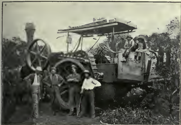
Clearing the Land for Grass.
