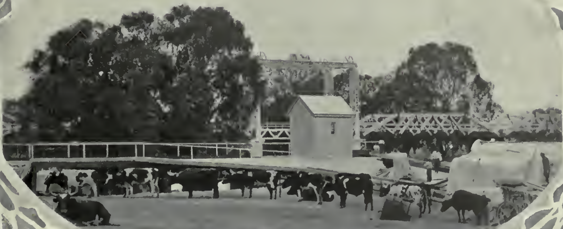
Wharf & Bridge Wentworth
