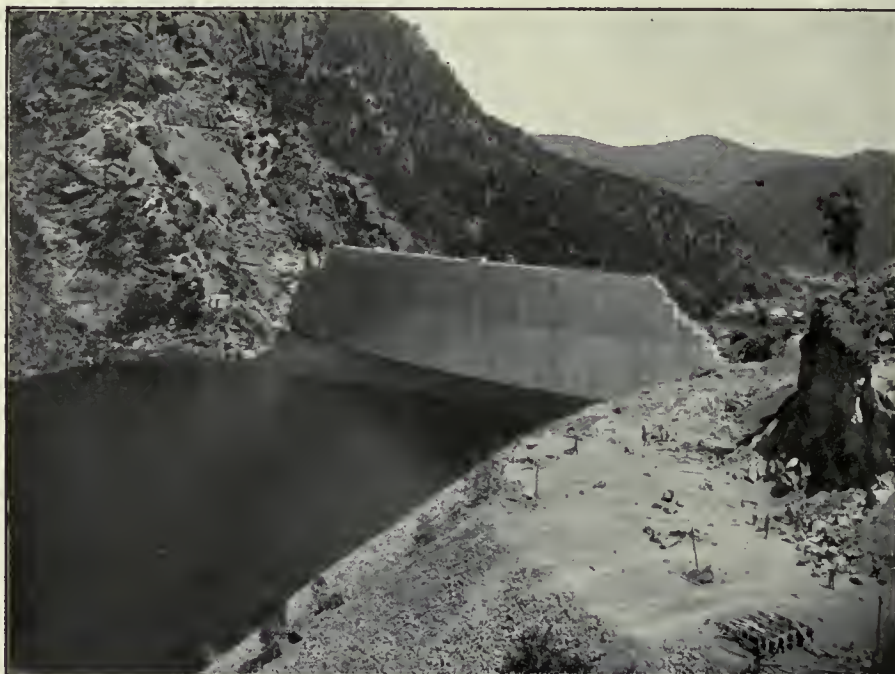
Burrinjuck Dam. Almost Completed (Up-stream Face)
