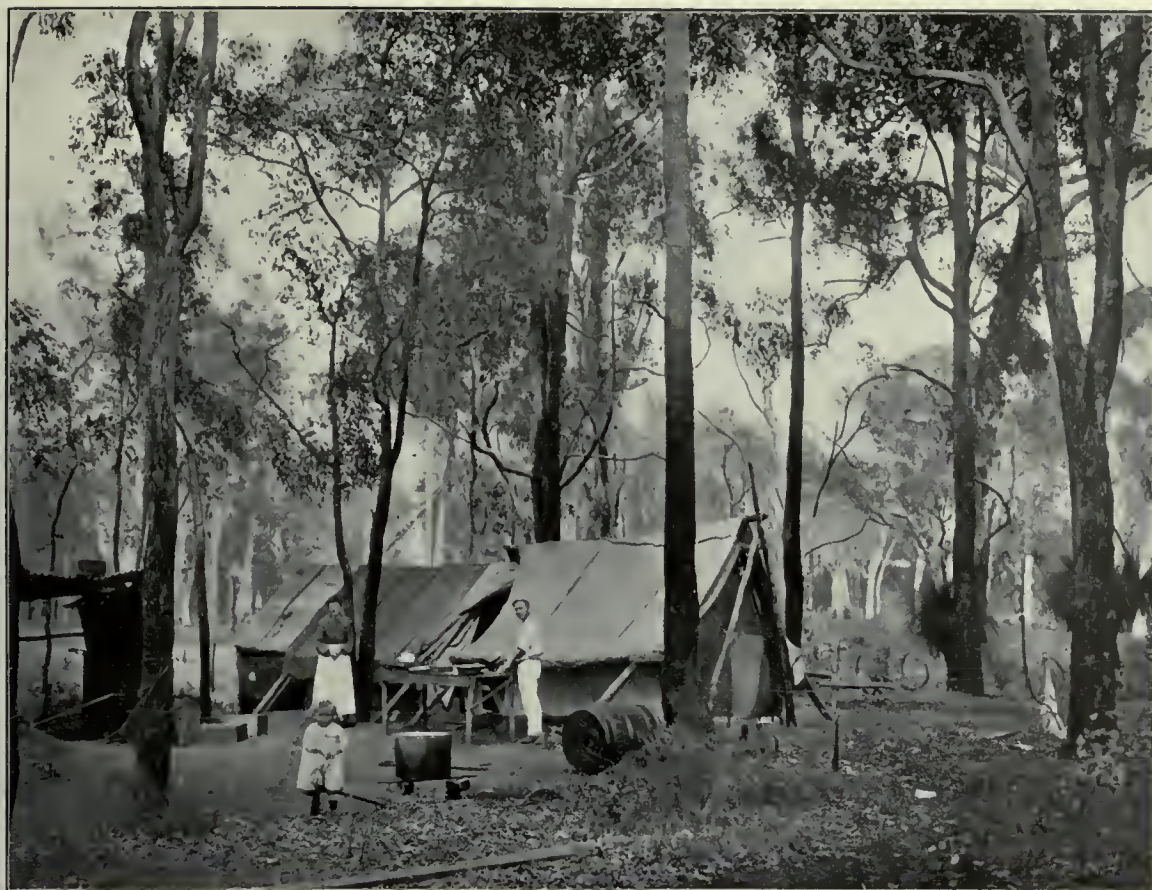
A New Selector at Brunswick
