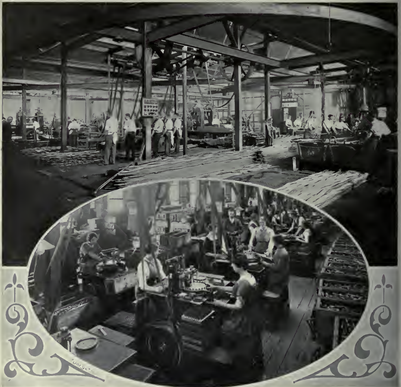
Interior of Metal-Rolling Mills
