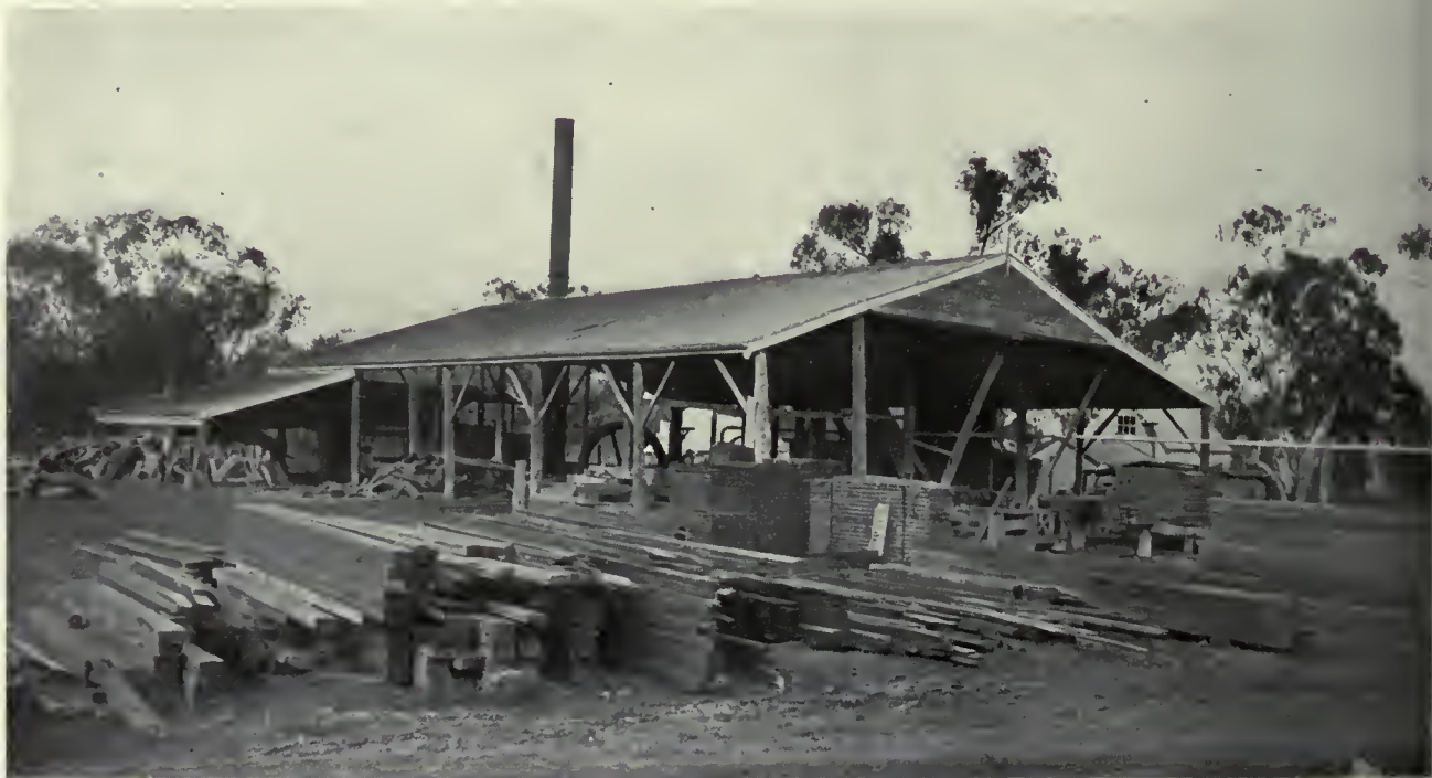
Sawmilling Plant, North Yanco Station
