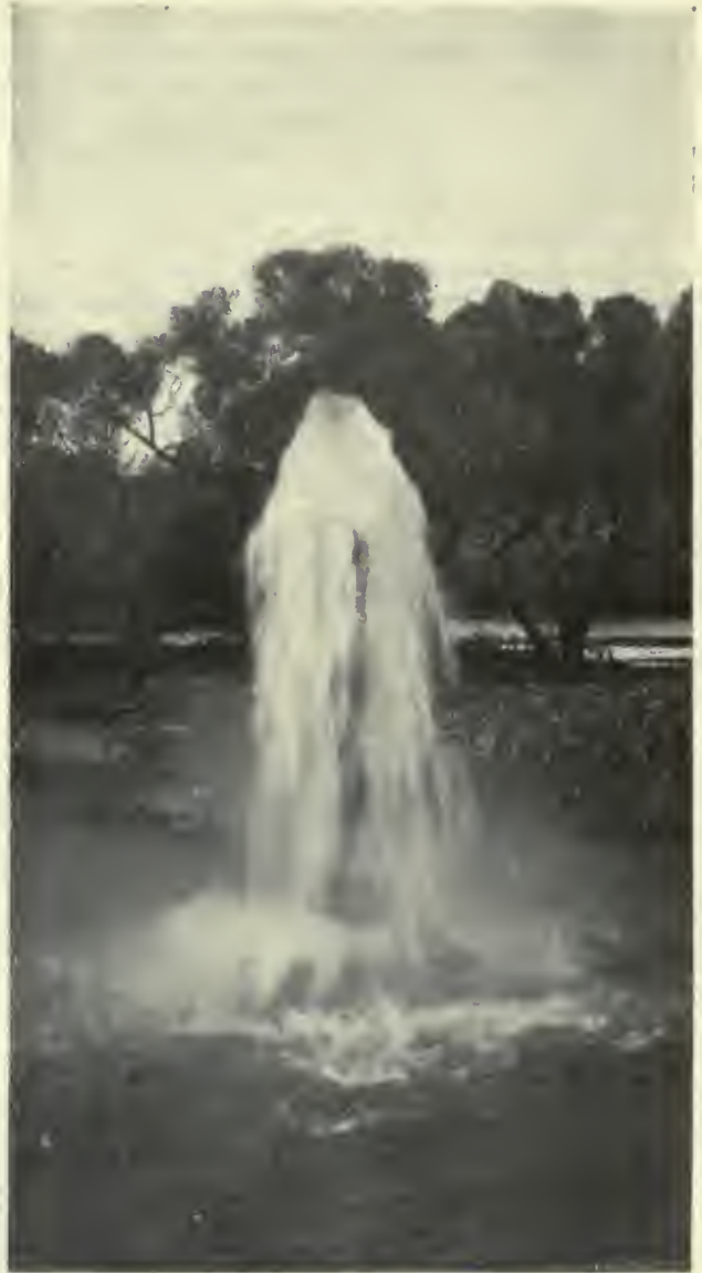
Artesian Bore, Allandale Station
