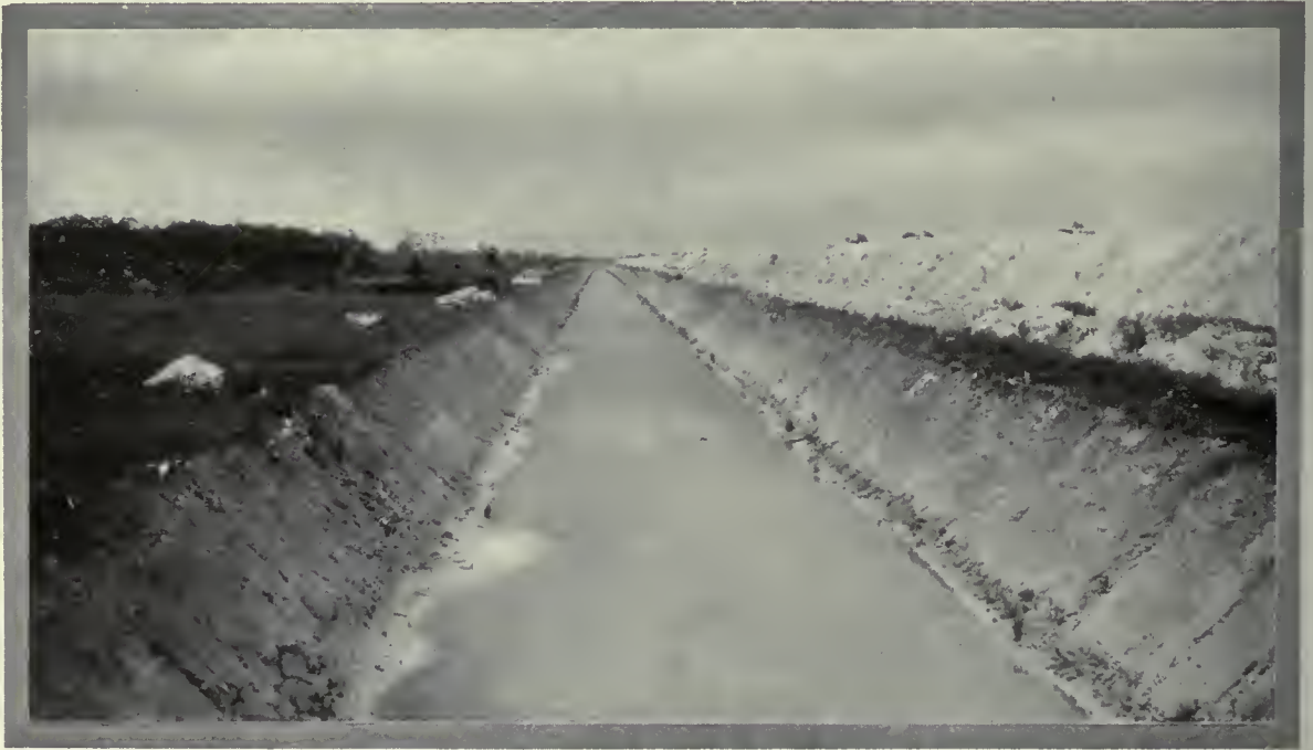
Drain excavated by machinery in limestone country
