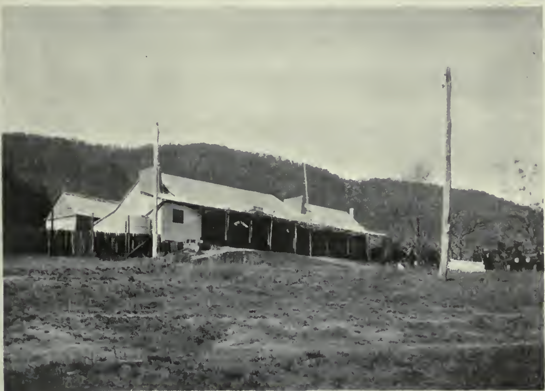
HALF-WAY HOUSE AT THE FOOT OF THE RANGE BUILT OF CEDAR, IN THE CEDAR COUNTRY.
