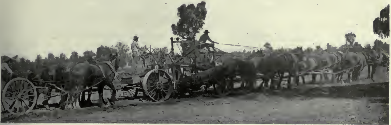
Era Grader, making Drains, Upper Yanco Station
