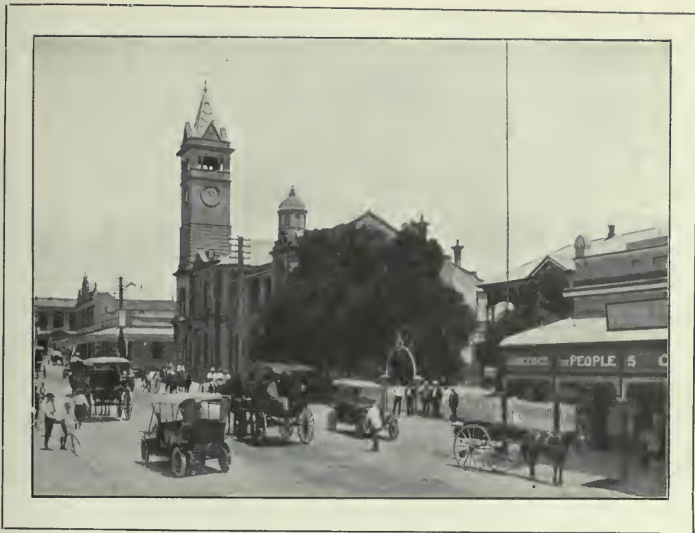
Gill Street, Charters Towers
