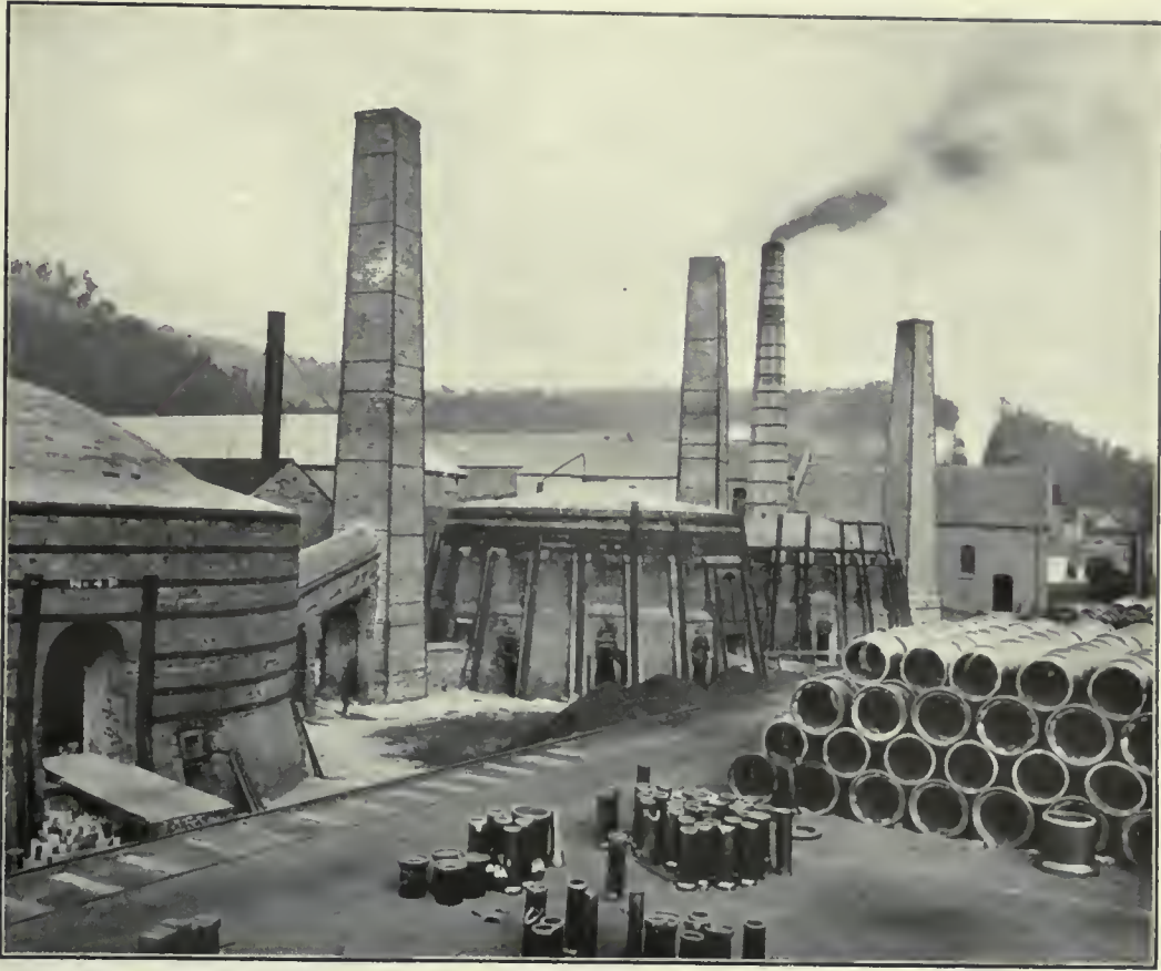
Brick and Drain-Pipe Works, Lithgow, N.S.W.
