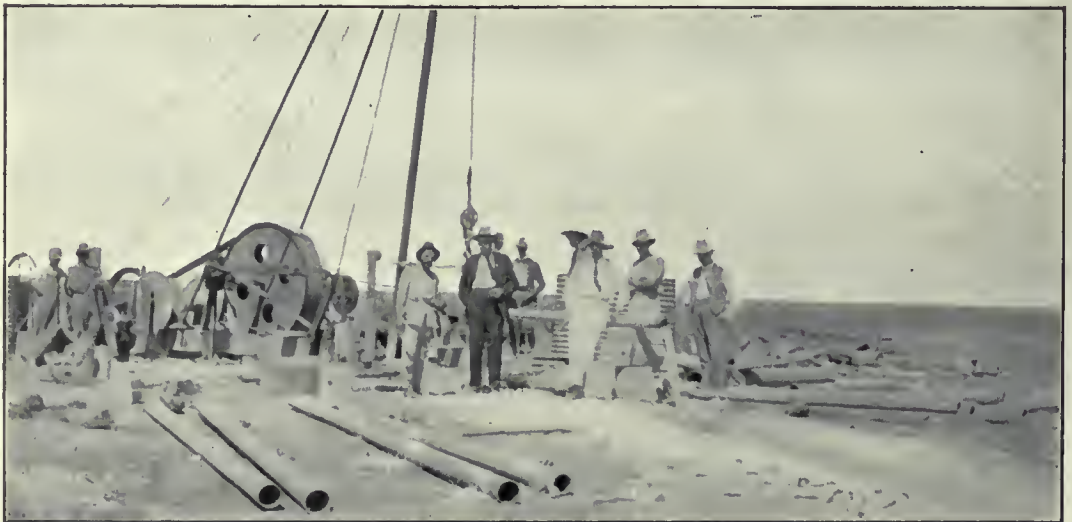
Freshwater Bore, West End of Railway
