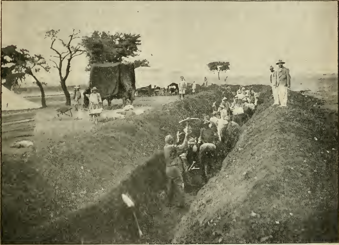
MAFEKING: NATIVES DIGGING A TRENCH.
