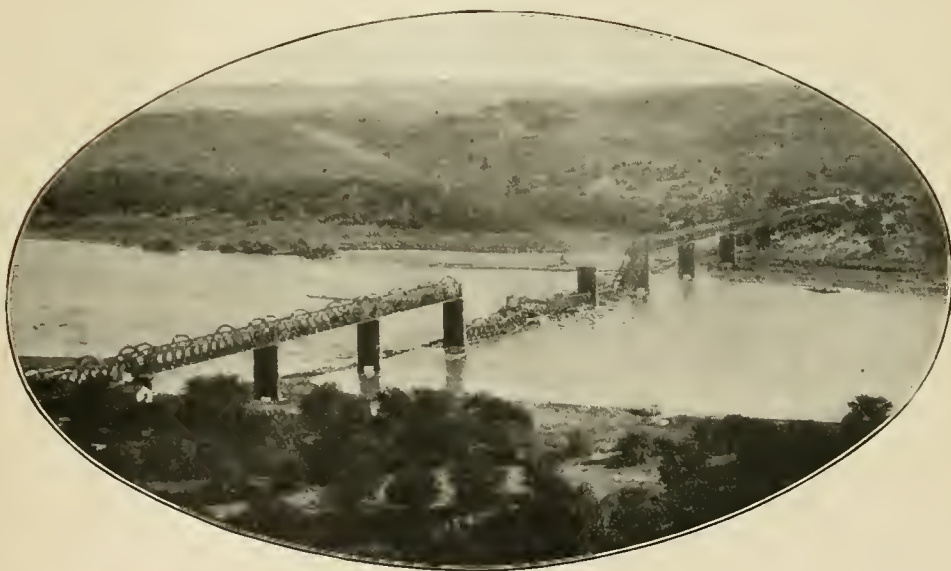
NORVALS FONT BRIDGE, AFTER ITS DESTRUCTION.
