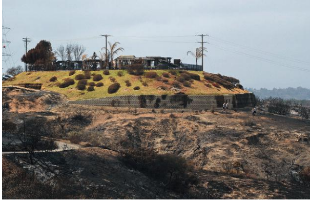
FIGURE 13.2 Homes burn because they are flammable. Many homes with adequate defensible space still burn in wildland fires because embers land on flammable materials around the home or enter through openings such as attic vents. These two homes burned during the 2014 Poinsettia Fire in Carlsbad, California, despite fire-safe landscaping, a firewall, and thinned wildland vegetation. Focusing exclusively on wildland vegetation clearing ignores the main reasons homes burn: they are flammable. (Photo credit: Richard W. Halsey.)
