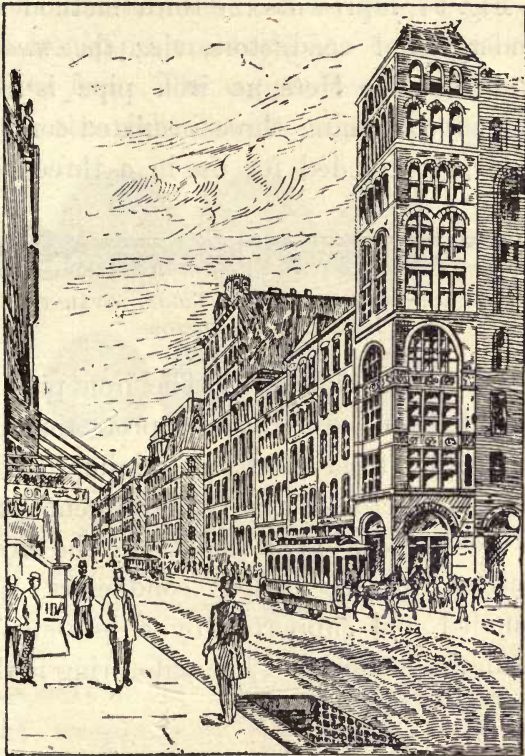
FIG. 96.—VIEW OF CITY STREET AFTER REMOVAL OF OVERHEAD WIRES.
