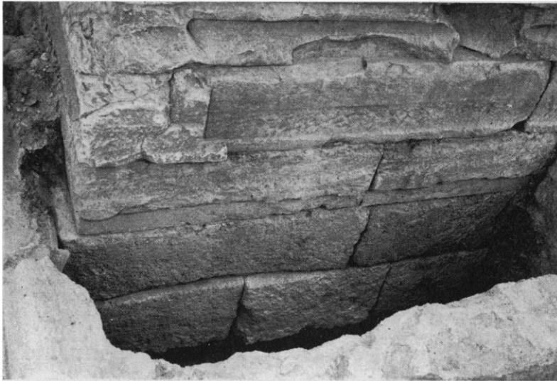
Fig. 15. Outer Corner of Foundation below Southwest Corner of Opisthodomos, from South
