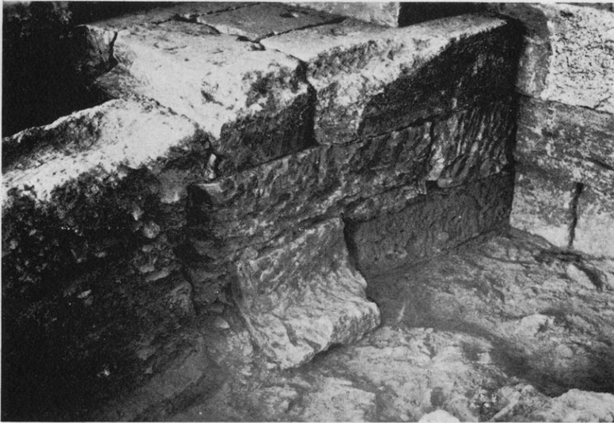
Fig. 28. Interior Column Foundations at Southwest Corner of Cella, with Earth Below
