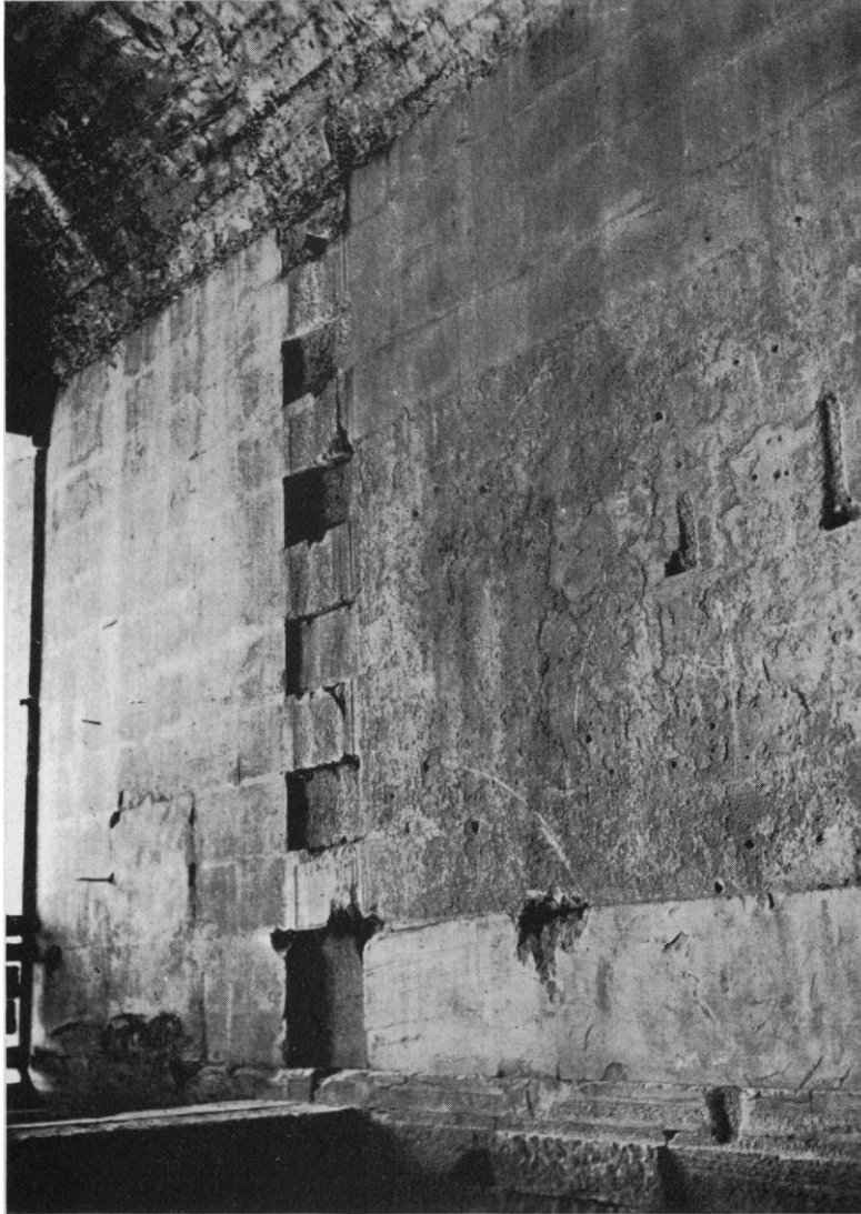
Fig. 31. South Wall of Cella at Junction with East Cross-Wall, Showing Mediaeval Plaster
