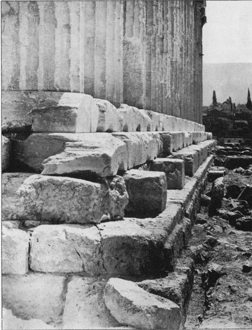
Fig. 12. South Foundation of the Hephaisteion, from West
