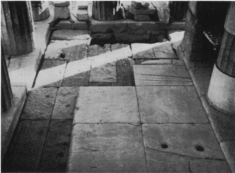
Fig. 24. Pavement and Underpinning of East Peristyle, from North
