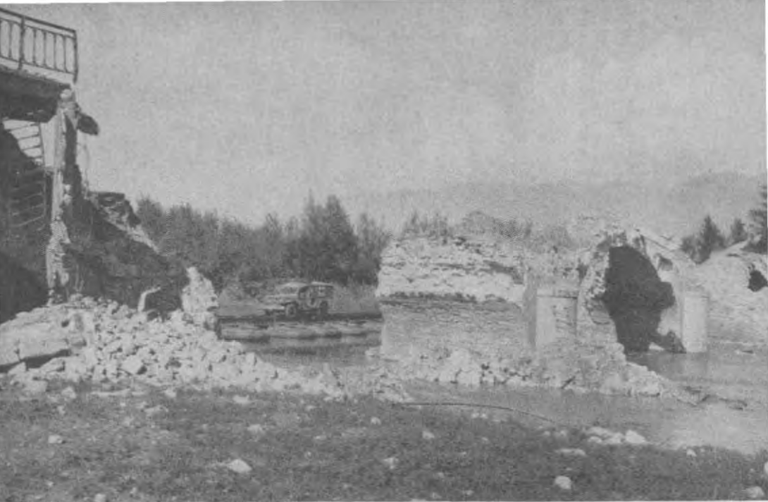
THE HIGHWAY BRIDGE ACROSS THE VOLTURNO on the road from Dragoni to Alife was blown by the Germans just before the 34th Division reached it. By 21 October trucks were crossing over the ponton bridge, seen in the center.
