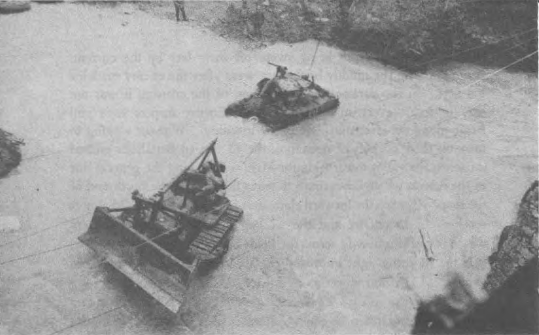
BULLDOZERS FERRIED TANKS ACROSS THE RIVER, cleared wrecked vehicles from vital roads, and improved bridge and ford sites. One bulldozer, working on the river bank, was fired on each time it showed itself; others had to give up operations because of enemy artillery attacks. The ponton bridge in the upper left corner of the picture had been constructed hastily for light traffic only.
