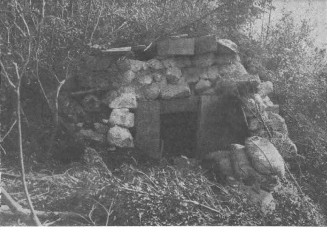
A GERMAN PILLBOX guards an approach to Mount Lungo. Machine-gun bunkers, mortar emplacements, and personnel shelters were made of local stone and in a setting of rock walls were invisible at a distance. Timbers and ties supported their overhead cover. Direct hits of heavy mortar shells did not penetrate them.
