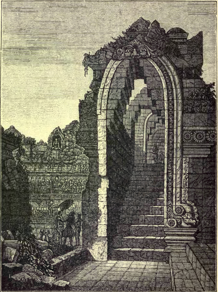
481. View of Central Entrance and Stairs at Boro-Budur. (From a Lithographic Plate.)
