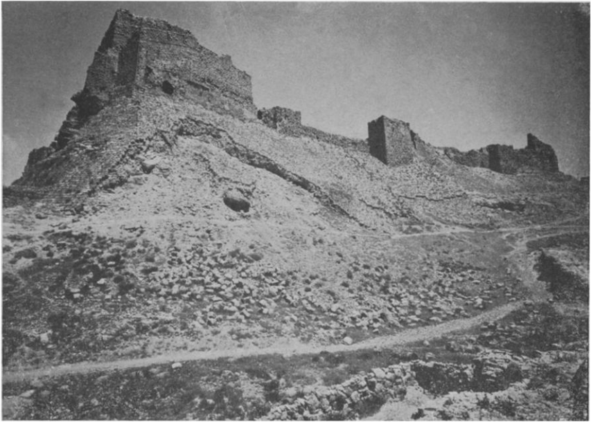
Fig. 11. Crusader castle of Kerak. View of the east side. (Photo Government of Palestine, Dept. of Antiquities.)
