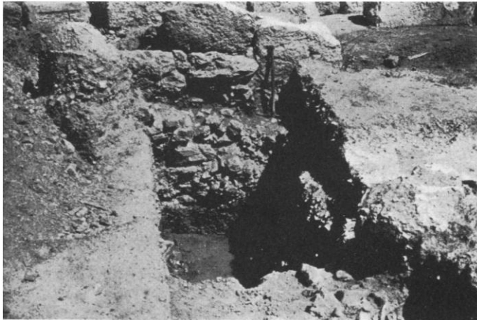
Fig. 6. Retaining Wall: Cut Across Road, showing 6th Century Packing and Polygonal Wall
