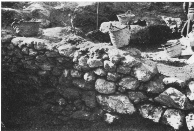
Fig. 4. Geometric Retaining Wall. Outer Face
