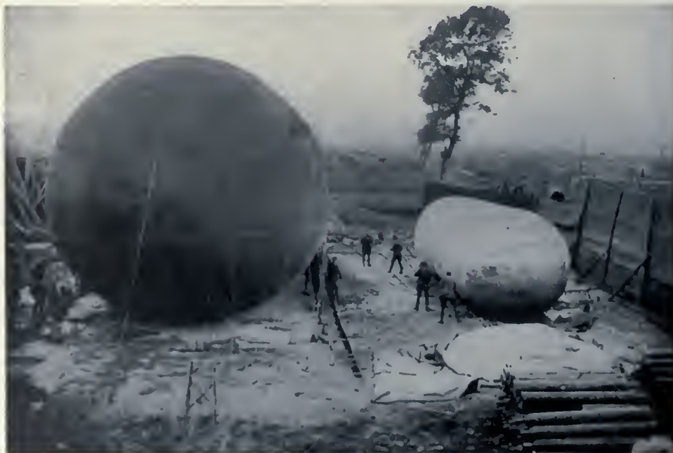
A Russian observation balloon and its "nurse." An observation balloon after inflation may stay in the air for an entire day without receiving additional gas. When it needs replenishing a smaller balloon, the "nurse," is brought up and the gas it contains is pressed into the larger balloon, the pressing being done by the men, who squeeze the "nurse."
