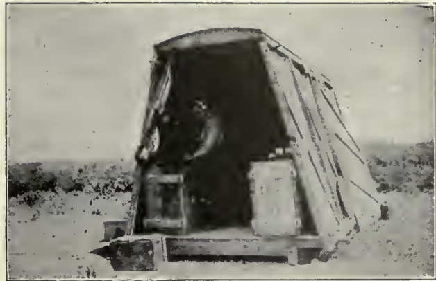
An improvised receiving station constructed with aeroplane packing boxes.
