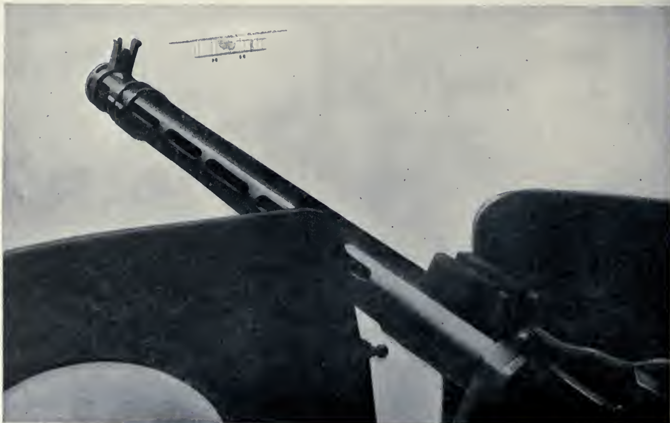
A 37 millimetre Hotchkiss cannon mounted on a French "Voisin" battleplane.
