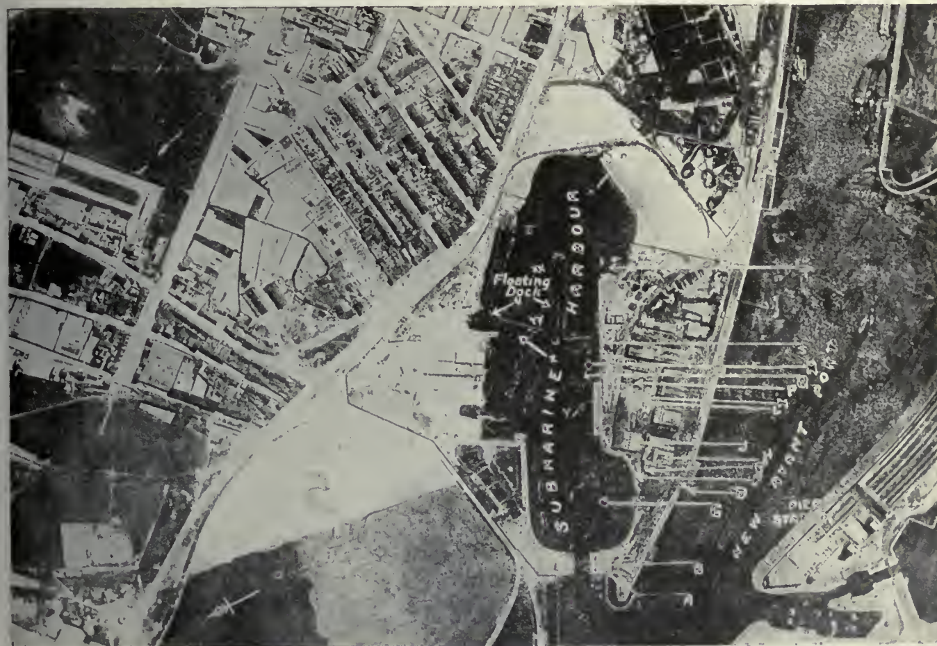
An official air-photograph of Ostend after the British naval bombardment. It will be seen that the bombardment was directed against the Germans' submarine lair, the letters indicating the principal hits. Thus B represents the damaged entrance gates to basin; C, Q and R, destroyers struck; D, U and Z, pier and jetties hit. The other letters indicate damage to the submarine harbor and adjacent buildings. Ostend is an important German naval base.
