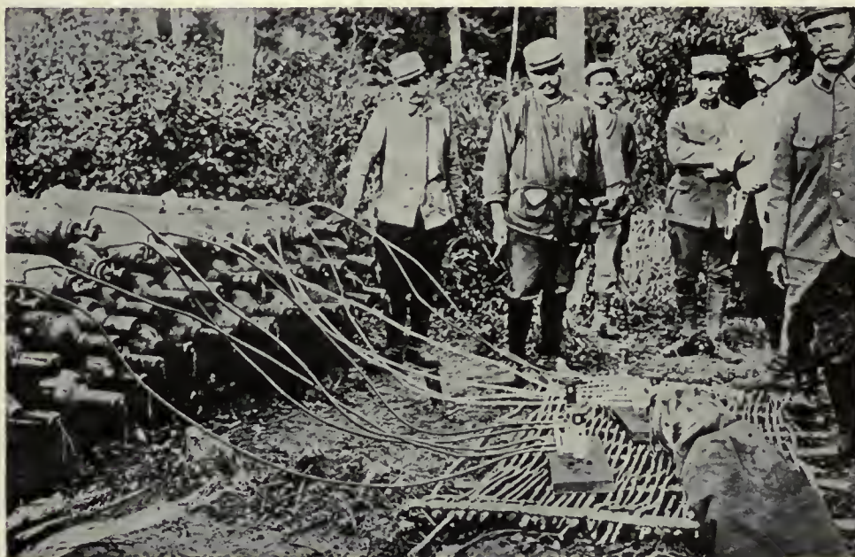
A battery of hydrogen gas cylinders attached to supply pipe of balloon being filled.
