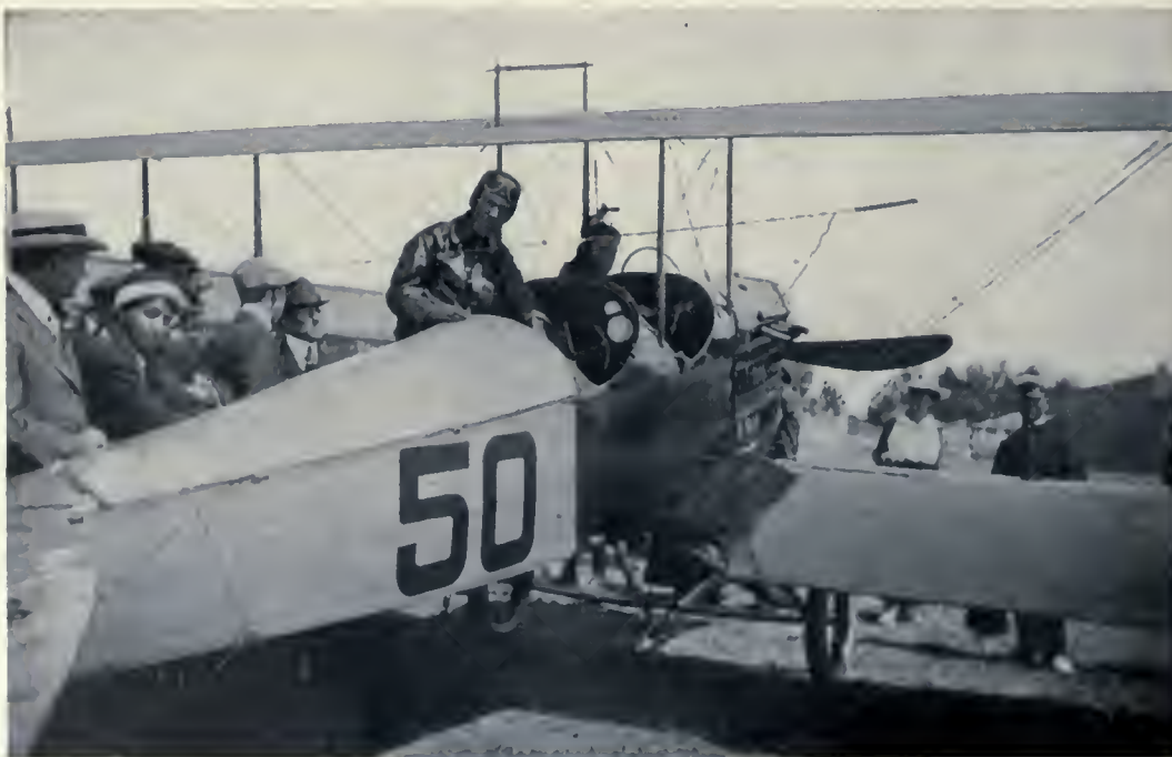
U. S. Army Aeroplane No. 50 of the North Island aviation school which was one of the aeroplanes which was equipped by Capt. C. C. Culver for radio work, the aerial wires being shown above the upper plane in the picture. Lieut. Herbert Dargue, U. S. A., is seen at the pilot's wheel, while Major Frank P. Lahm is in the observer's seat. The officers had just completed a flight.
