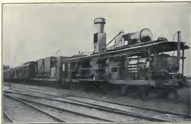
Portable hydrogen gas plant constructed for the chief engineering department of the Imperial Russian War Office.
