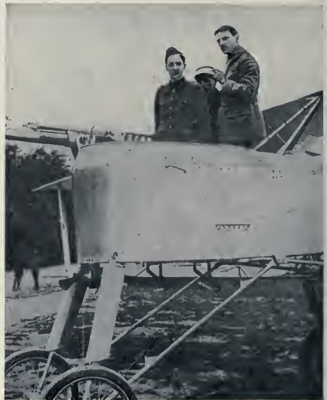
A 37 millimeter gun mounted on a Voisin-Peugeot gun plane.
