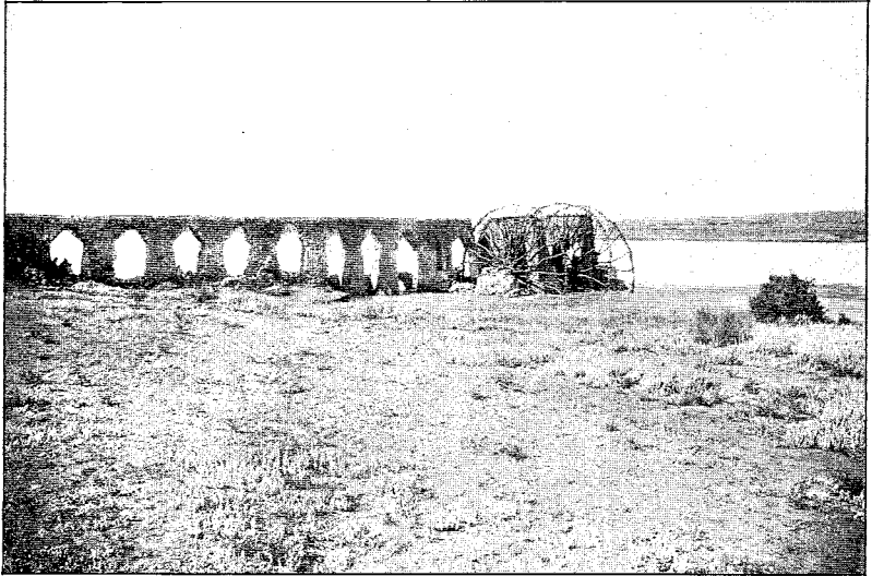
FIG. 9—Flush wheel, fields of al-Haffe.
