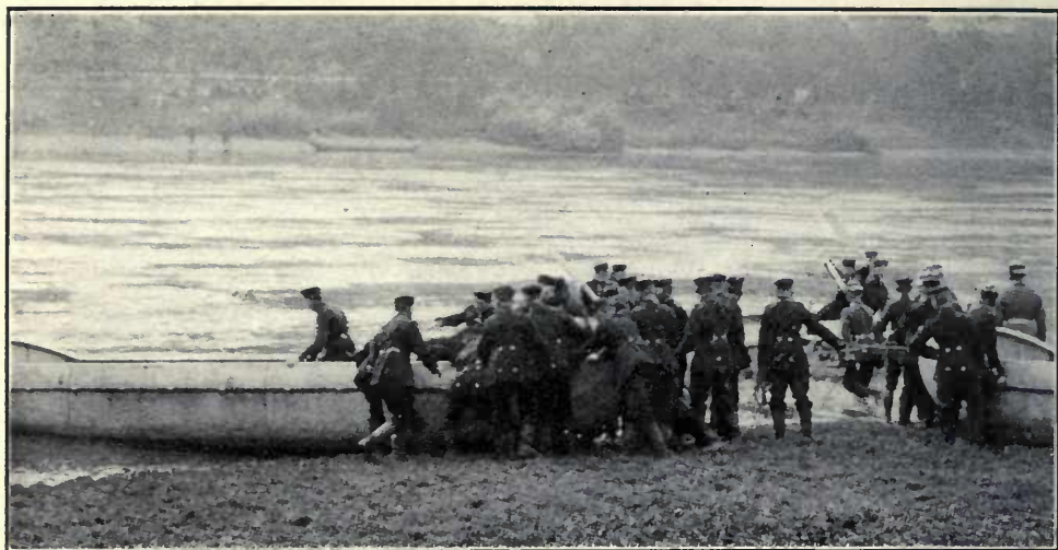
Floating the Pontoons
