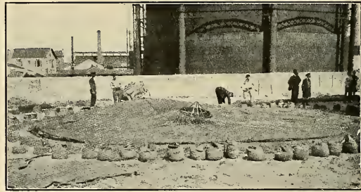
FIGURE 5 ARRANGING BALLOON PREPARATORY TO INFLATING
