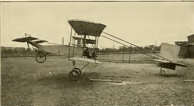
THE NEW RACING VOISIN BIPLANE FITTED WITH AN E. N. V. MOTOR: IT IS SAID TO FLY AT SIXTY MILES AN HOUR. THE USUAL VERTICAL PARTITIONS ARE REPLACED BY ALERONS.
