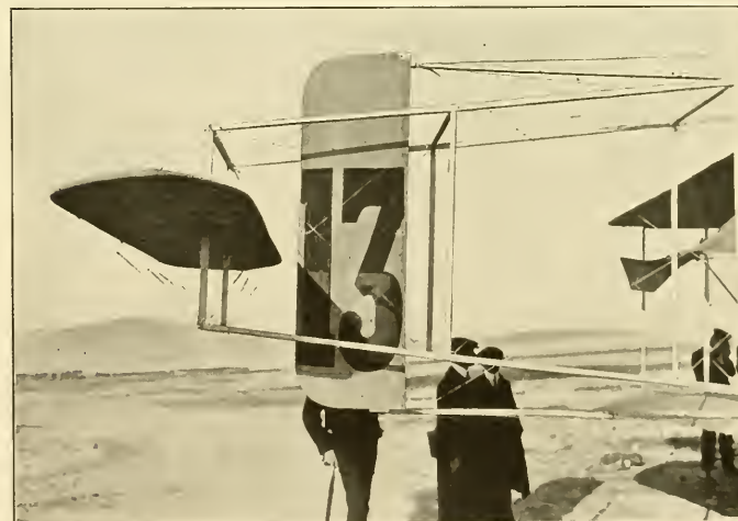
THE TAIL OF THE SHORT-WRIGHT BIPLANE, USED BY THE HON. C. ROLLS, AT NICE, SHOWING THE ADDITION MADE BY THE ENGLISH BUILDERS TO THE ORIGINAL WRIGHT DESIGN, OF A FIXED HORIZONTAL SURFACE AT THE REAR.
