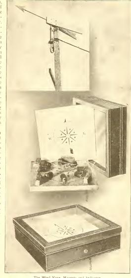
The Wind Vane, Magnets and Indicator
