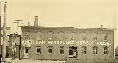
FRONT VIEW OF THE AMERICAN AEROPLANE SUPPLY HOUSE'S NEW FACTORY AT HEMPSTEAD, LONG ISLAND.
