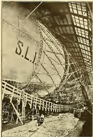
The rigid airship "Schuette-Lanz I (Zeppelin type)" in process of construction by the German Air Navy League, and now used in the German Army. Note the fine engineering displayed in the construction of the wooden ribs and metal bracing which is all socketed to withstand collisions.
