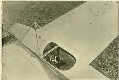
Heinrich 1912 Mono-Biplane, Model (A) showing seat, also windows in side and bottom
