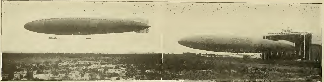
Pictures 9 and 10 show on the right the Schuette-Lanz airship leaving its hangar, and on the left the same dirigible starting off on a test flight. The picture on the left shows clearly the position of the under-hanging cars which as can be noticed are not rigidly attached to the hull but simply hang loosely from it. Attention is also called to the streamline shape of the hull which, in spite of the underhanging cars, allows the airship to attain a speed of 42 miles an hour.
