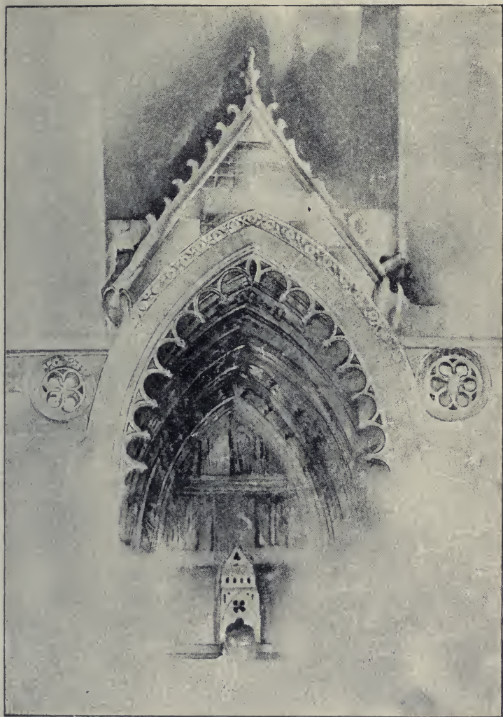
PLATE II.—THE BIBLE OF AMIENS. NORTHERN PORCH BEFORE RESTORATION.
