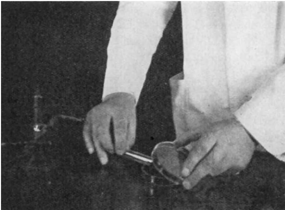
FIG. 4.—Petri dish and the method of pouring a plate
