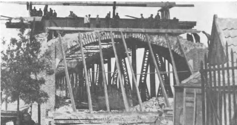
4. The Münsterwalde Bridge being dismantled by the Poles.
