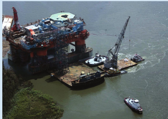
Hurricane Katrina in August 2005 damaged several oil platforms operating in the Gulf of Mexico and thus caused a temporary reduction in the supply of oil.
