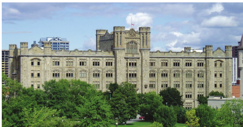
The Canada Revenue Agency, with headquarters in the Connaught Building in Ottawa, is the government department that collects all federal tax revenues in Canada.
