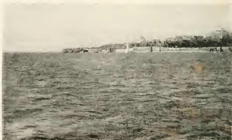
THE SOUTHEAST SEA WALL
