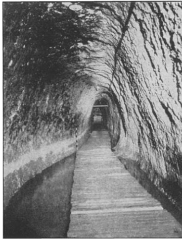
Fig. 6. A monument to Hebrew engineering: part of the ancient Megiddo water system. Lack of water within the walls of Megiddo, city of continual strife and the marching ground of many armies, would have rendered it powerless to withstand siege. Consequently, a cave-well, quite outside the city wall, was connected by means of this more than one hundred and fifty foot tunnel to a shaft sunk inside the wall. By an amazing feat of engineering skill, tunnelling proceeded from both ends at the same time (from the vertical shaft as from the well), as it did at the famous tunnel of Siloam. (Oriental Institute, University of Chicago)
