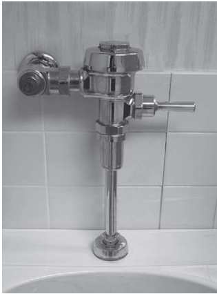
flushometer (flushometer valve)
