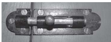
barrel bolt (tower bolt)
