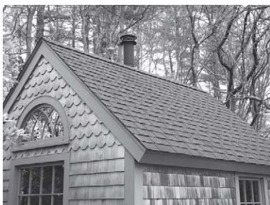
asphalt shingles (composition shingles, strip slates)
