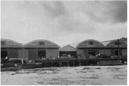
Abb. 42. Kaianlage der East Asiatic Company.
