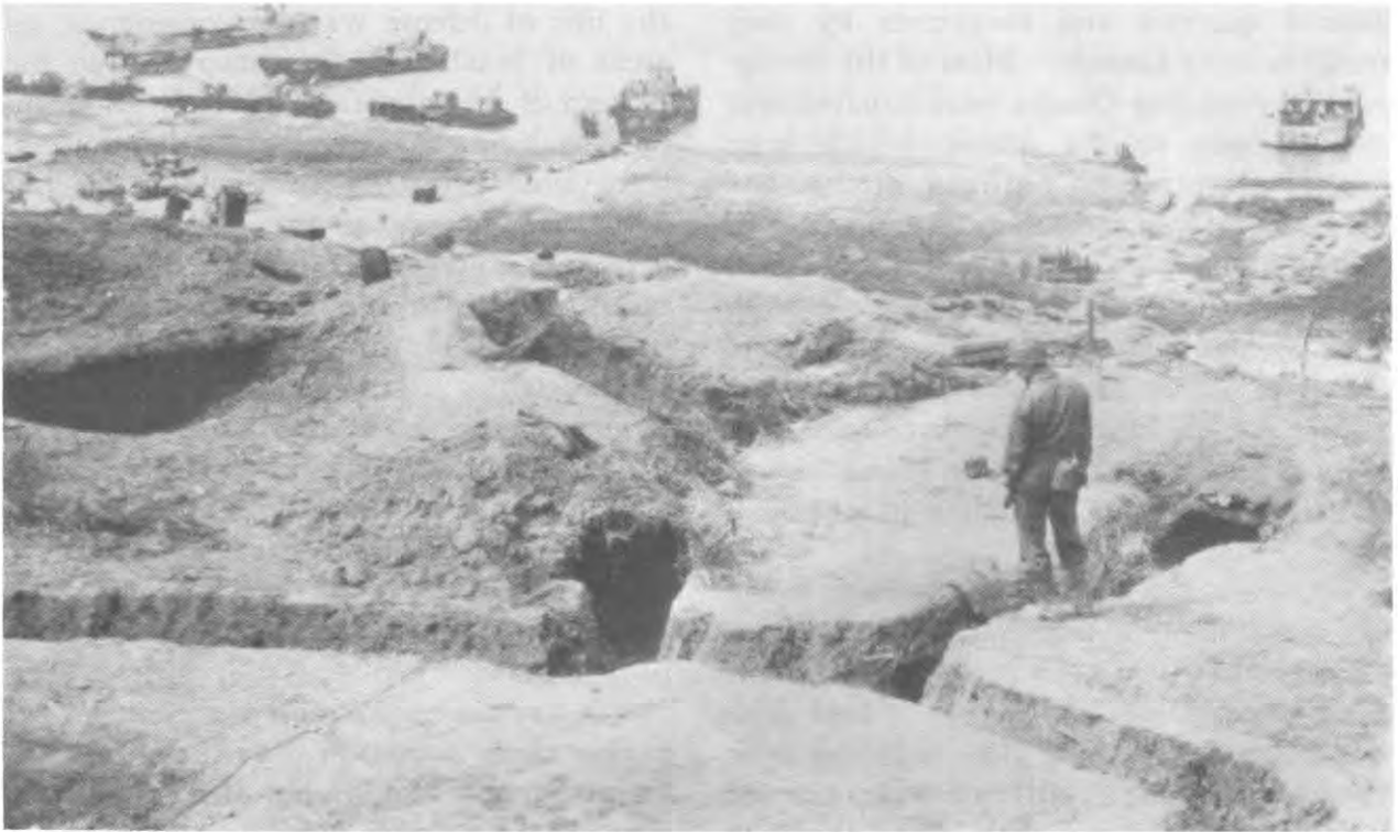
TRENCHES ALONG THE BLUFF EDGE were the main German defenses between strongpoints guarding draws. These trenches, leading from dugouts to firing positions, overlooked Easy Red Beach west of E-1 draw. Such systems usually included machine-gun positions.
