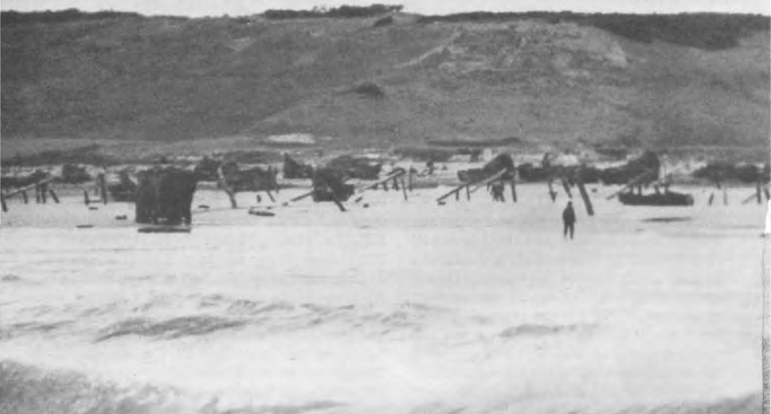
E-1 STRONGPOINT, to the west of the draw, was neutralized by a boat team of Company E, 16th Infantry, which came on it from the woods to the rear. The photograph above, taken a day later, shows beach obstacles and wreckage along the top of the tidal flat.
