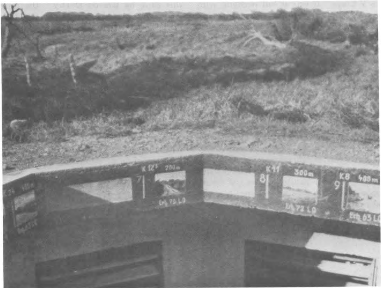
GERMAN MORTAR POSITION, in the strongpoint on the bluff just west of Vierville draw, looking inland. The gunners had oil-painted panoramic sketches of ground features near the position, with ranges and deflections for hitting more important target areas.
