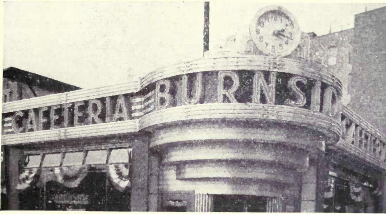
FIG. 29.—Outline skeleton sign applied as a triple-tube unit.
