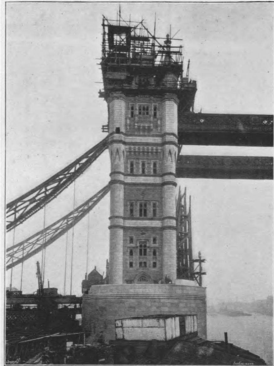
Fig. 80—THE NORTHERN MAIN PIER—MASONRY SUPERSTRUCTURE, NOVEMBER, 1893
