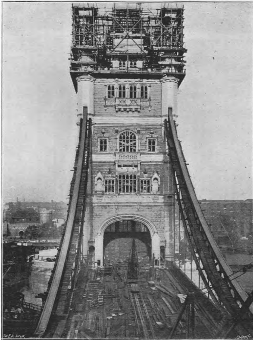
Fig. 79—THE SOUTHERN MAIN PIER MASONRY SUPERSTRUCTURE, OCTOBER, 1893
