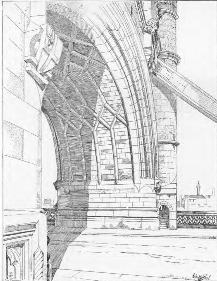
Fig. 83—MASONRY ARCH OVER NORTHERN ABUTMENT
