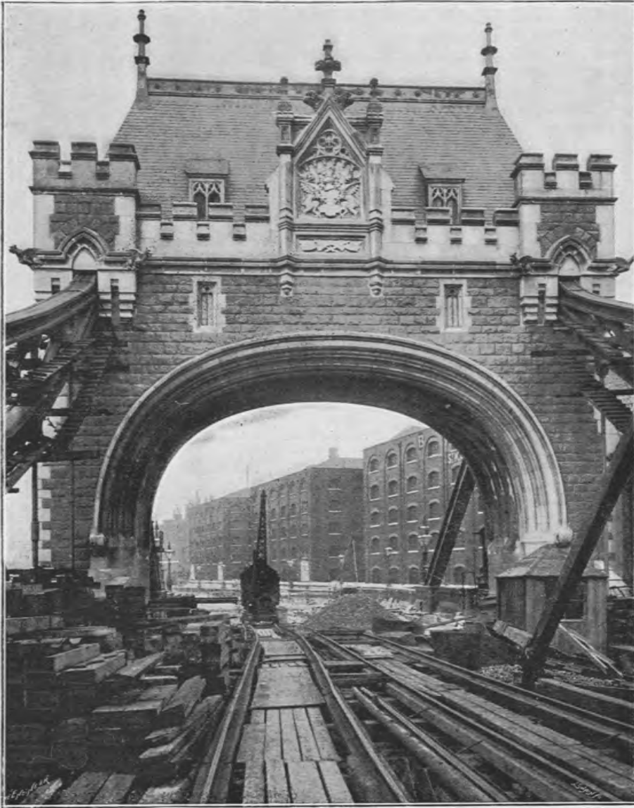
Fig. 82—FRONT ELEVATION OF MIDDLESEX ABUTMENT
