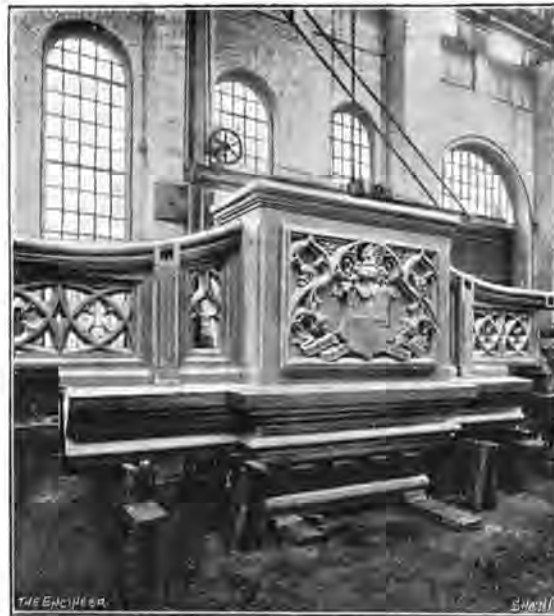
Fig. 61—CENTRAL PANEL, SIDE SPAN PARAPETS
