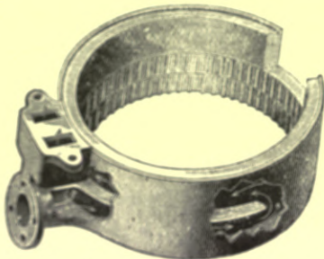
Fig. 512.—View of Fire-pot of the "Oxford" Boiler, showing circulation of water.
